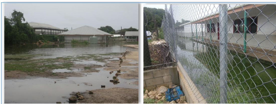
Figure III-IV Fence foundations obstruct flow of water to drainage system
