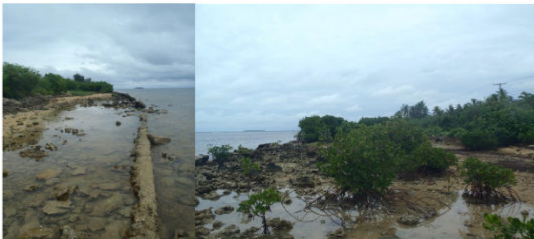
Figure 18: Failed seawall looking west to Manuka (left) and mangrove stands behind failed seawall
