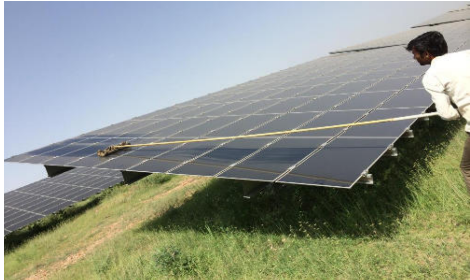
Photograph showing cleaning of PV panels
