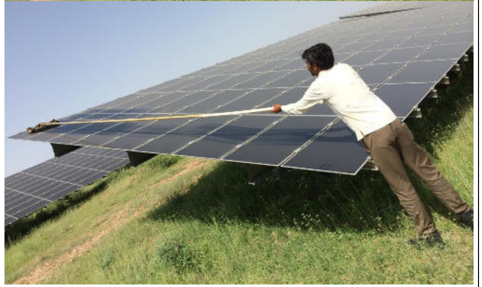
Photograph showing cleaning of PV panels
