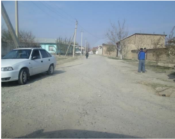
Pic. 3. Khalkobod street where sewerage pipes will be laid in the middle of the mahalla street.
