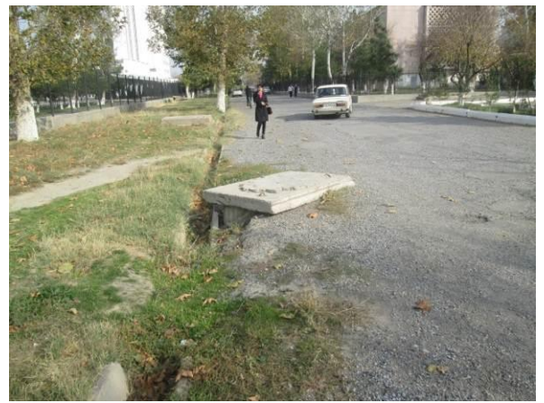
Pic.8. Near Firdavs hospital where sewerage pipes will be rehabilitated along the street
