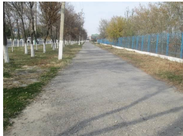
Pic. 2. Pipes will be laid in the middle of the sidewalk. Tashkentskaya street
