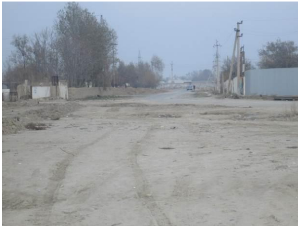
Pic. 5. Tukimachilik street where sewerage pipe will be laid in the middle of the street.
