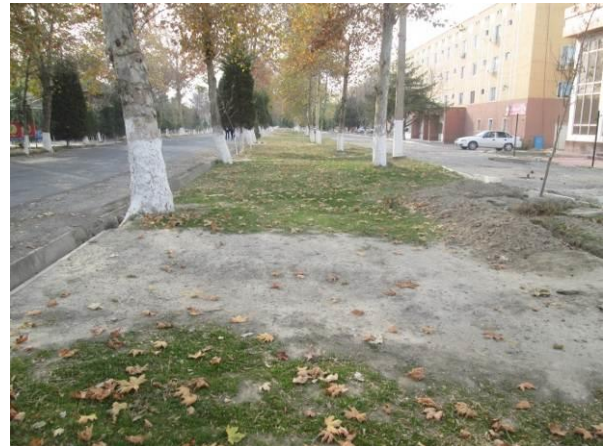
Pic. 6. Bulvarnaya street where sewerage pipe will be laid in the middle of the alley.
