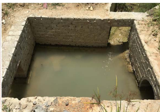
Pic.2 On-site Settling Tank of Construction Wastewater (Taken in July 2016)
