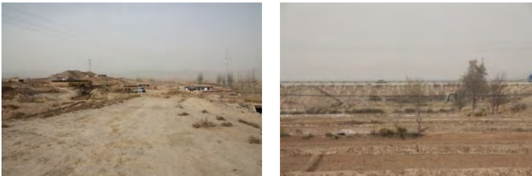
Figure 2-1: Site Existing Condition of Xihuan Road
