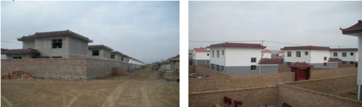
Figure 6-3: Resettlement Houses under Construction in LIP Resettlement Living Area (November 2013)
