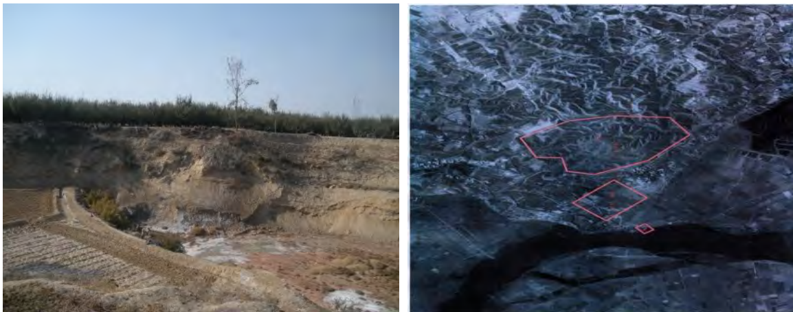
Figure 2-2: Site Existing Condition of 1 st WSP (Left) and Layout of the Pumping station, the 1 st WSP and the Sludge Landfill Site (Right)
