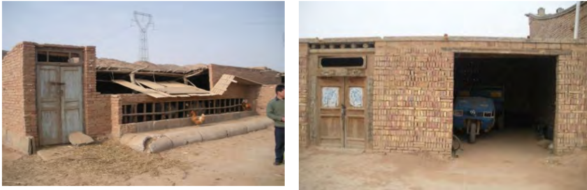
Figure 2-6: Affected Auxiliary Structures—Chicken Home and Simple Storage Shed
