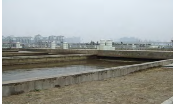
Fig. 2: Oxidation ditch with brush aerators (phase 1 plant)
