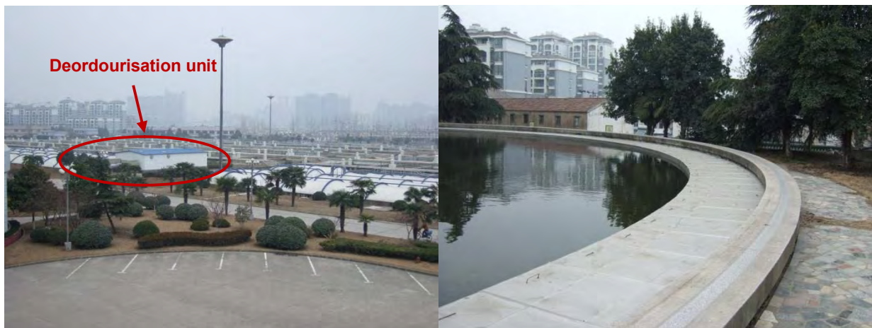
Fig 5: Covered anaerobic tanks and de-odourisation unit (left), covered clarifier (right)
