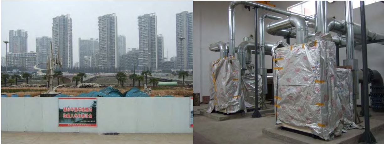
Fig 6: Modification works at Phase 2 oxidation ditches (left), new ABS magnetic bearing air blower (right)
