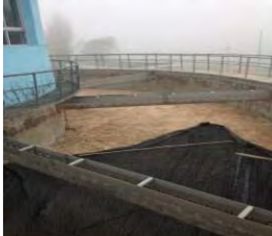
Lamella Mechanical Sedimentation Tank
