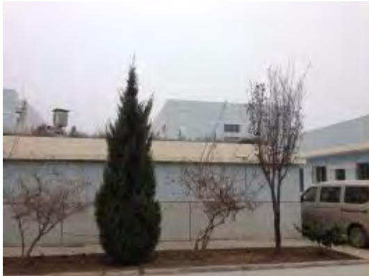
Clean Water Tank
