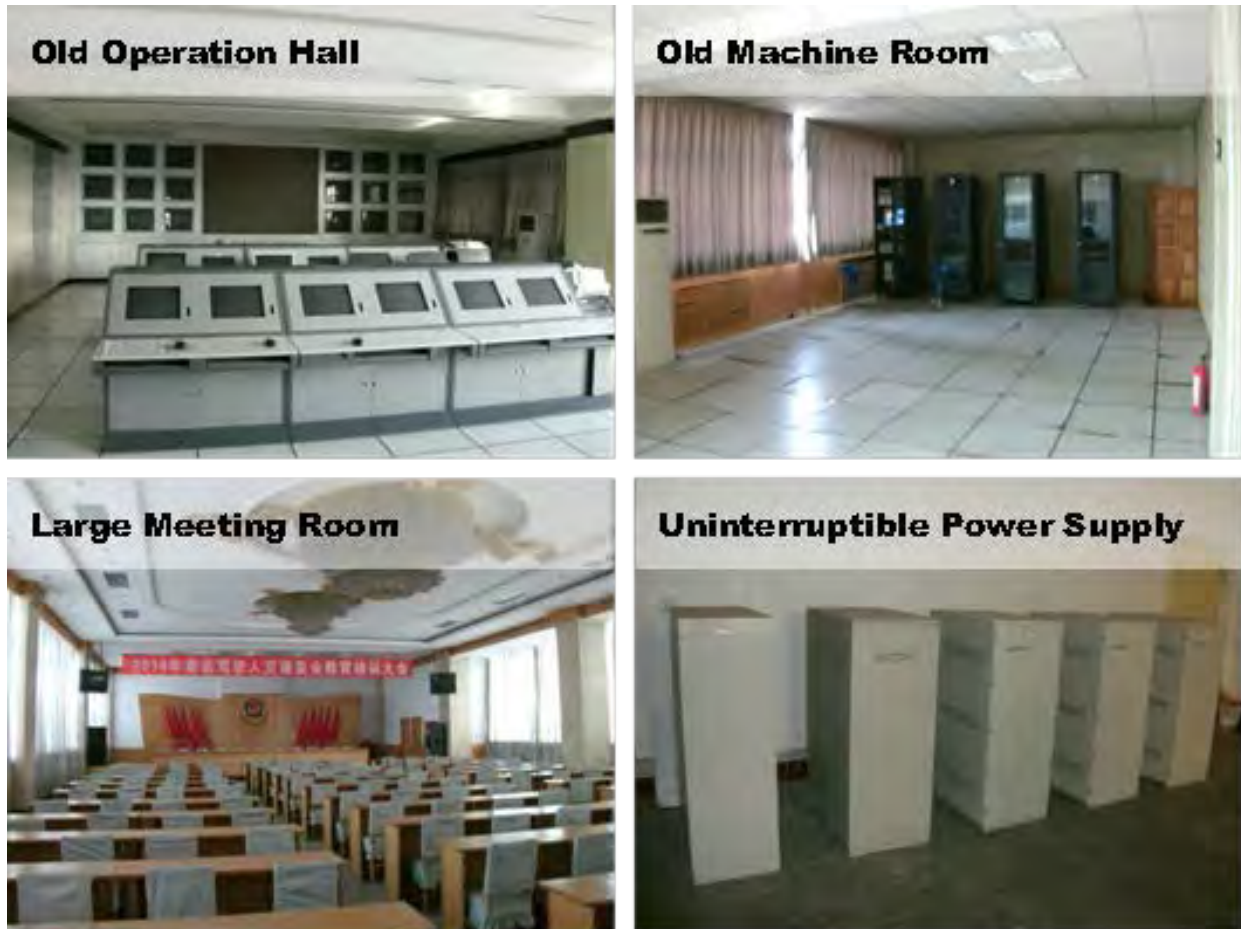
Figure 11: Existing traffic police operation center infrastructure and facilities
