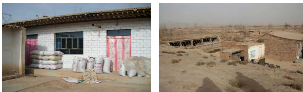
Figure 2-5: Rural Residential Houses to Be Demolished
