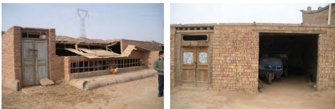
Figure 2-6: Affected Auxiliary Structures—Chicken Home and Simple Storage Shed
