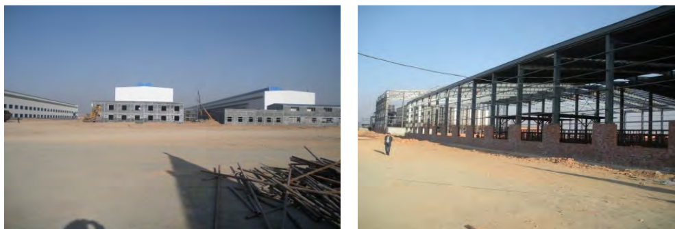
Figure 6-1: Gansu Hongtai Aluminum Co. (left) and Gansu Kaisi Ceramic High Quality Wall Bricks (right) (December 2013)
