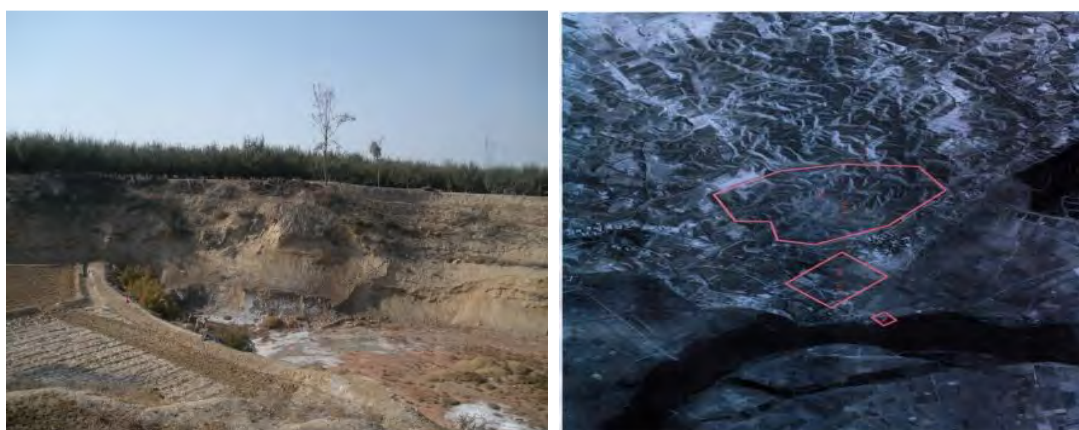
Figure 2-2: Site Existing Condition of 1 st WSP(Left) and Layout of the Pumping station, the 1 st WSP and the Sludge Landfill Site (Right)
