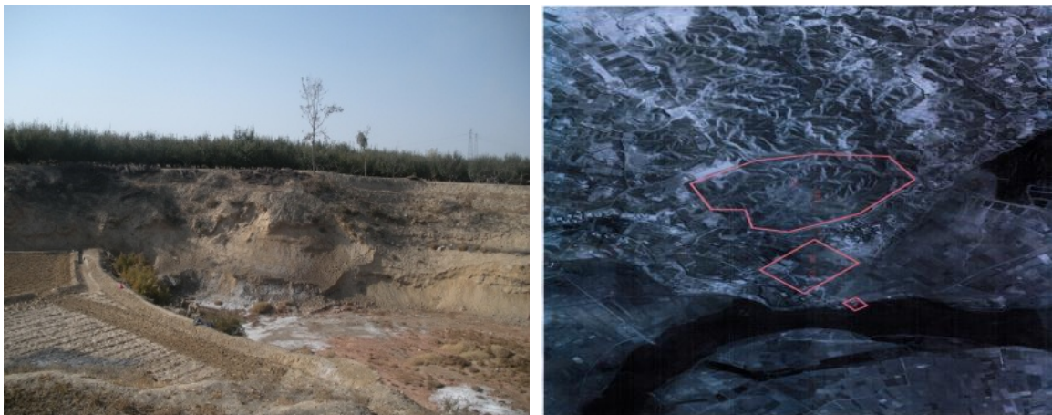
Figure 2-2: Site Existing Condition of 1 st WSP (Left) and Layout of the Pumping station, the 1 st WSP and the Sludge Landfill Site (Right)
