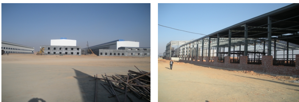
Figure 6-1: Gansu Hongtai Aluminum Co. (left) and Gansu Kaisi Ceramic High Quality Wall Bricks (right) (December 2013)
