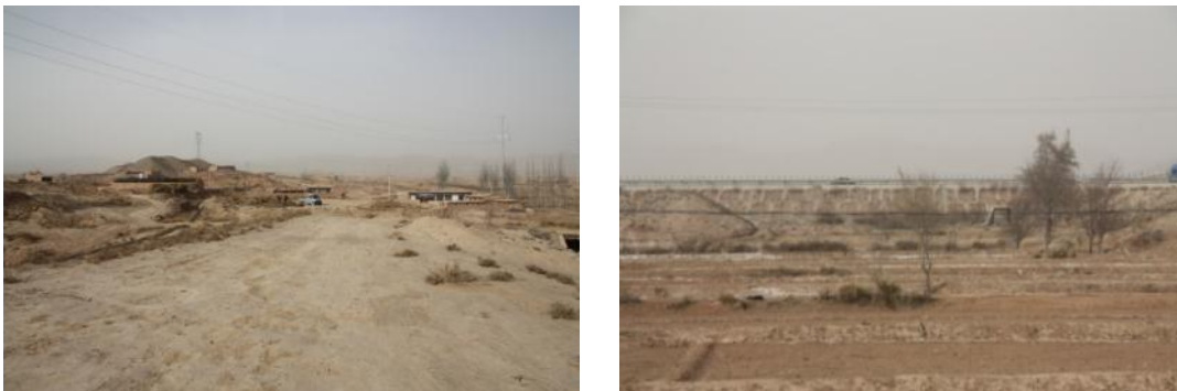
Figure 2-1: Site Existing Condition of Xihuan Road
