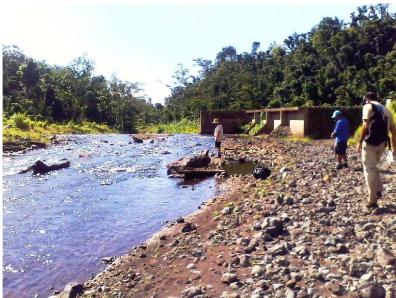
Plate 9. The damaged headpond and intake on the Samasoni HPP in the lower Vaisigano river valley. Photo by Moetuasivi F Asiono.
