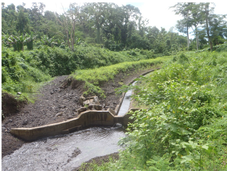
Plate 6. The Alaoa HPP Western Intake. Note the whole river flow going into the headrace. Photo by James Atherton
