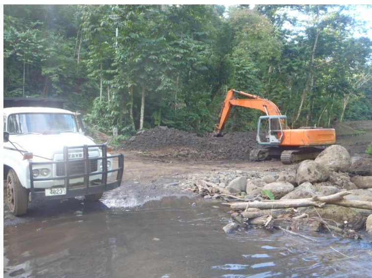
Plate 2. The Samoa Water Authority is currently dredging silt from the reservoir causing significant siltation downstream. Upstream from this point the river is stagnant and has large number of invasive Livebearers present ( Poecilia Mexicana ). Photo by James Atherton.
