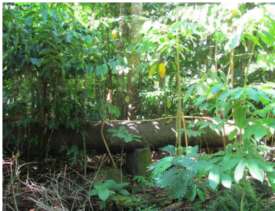
Figure 18: Existing penstock overgrown by rubber trees
