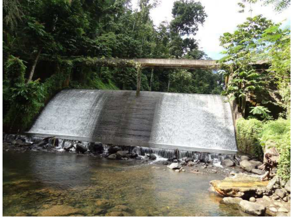
Figure 4: The spillway at the existing dam
