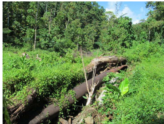
Figure 7: Existing, damaged penstock
