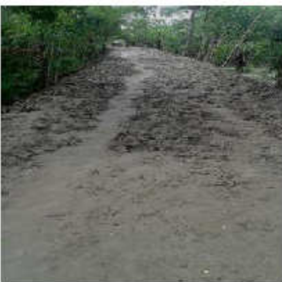
Re-sectioning of Coastal Embankment
