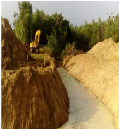
Excavation of khal heaping spoil earth on the Banak
