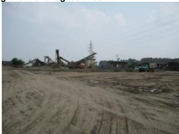
Plate III.1: Existing port with sand and gravel handling facilities
