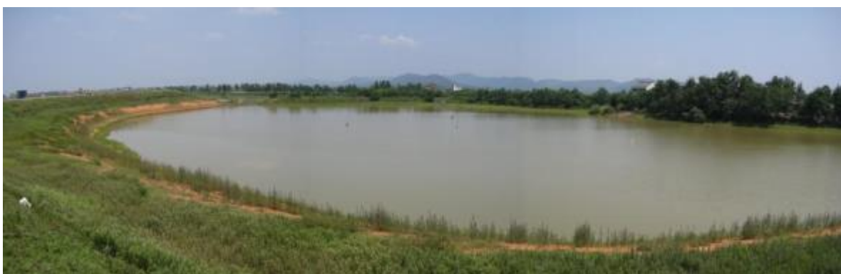
Plate III.20: Proposed dredged dumping site in pond within Shuiyang River flood bunds
