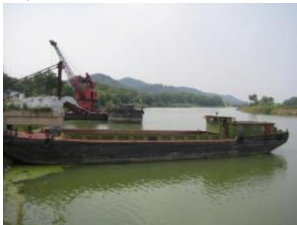
Plate III.2: Existing port on the Shuiyang River
