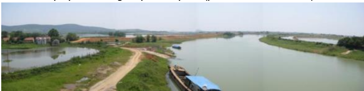
Plate III.19: View upstream of the Shuiyang River, new Flood Alleviation Channel and proposed dredged spoil dump site (pond in middle distance)
