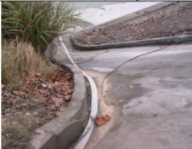
Drainage ditch in asphalt mixing station
