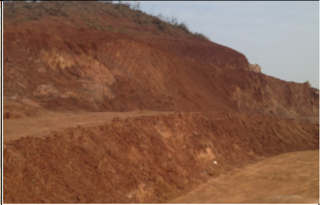
Terraced soil excavation to minimize soil erosion
