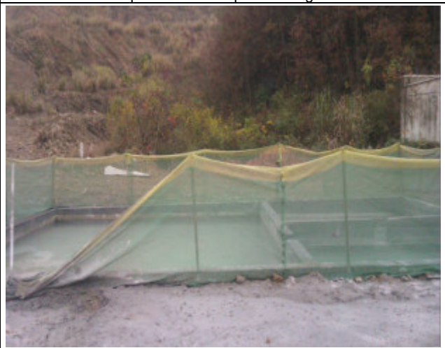
3-chamber sedimentation tank in NO2-2 asphalt mixing station
