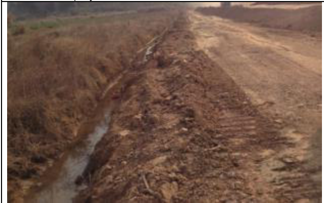
Temporary drainage ditch during subgrade works to minimize soil erosion
