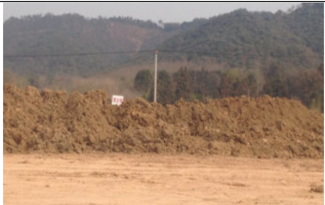
#2 spoil disposal site at K6+300
