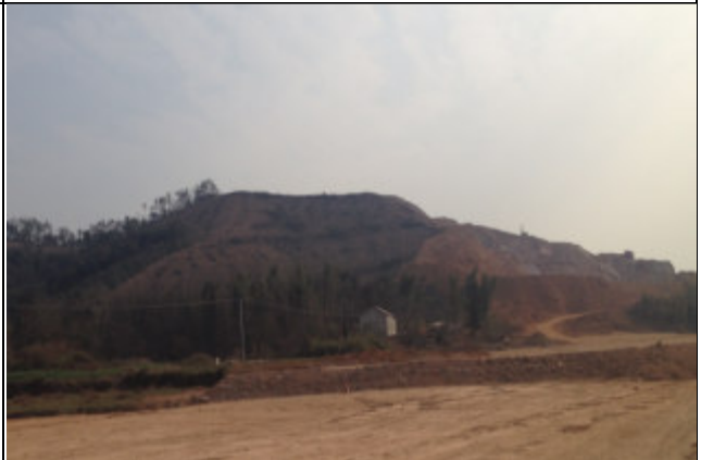
#2 borrow area at K6+800
