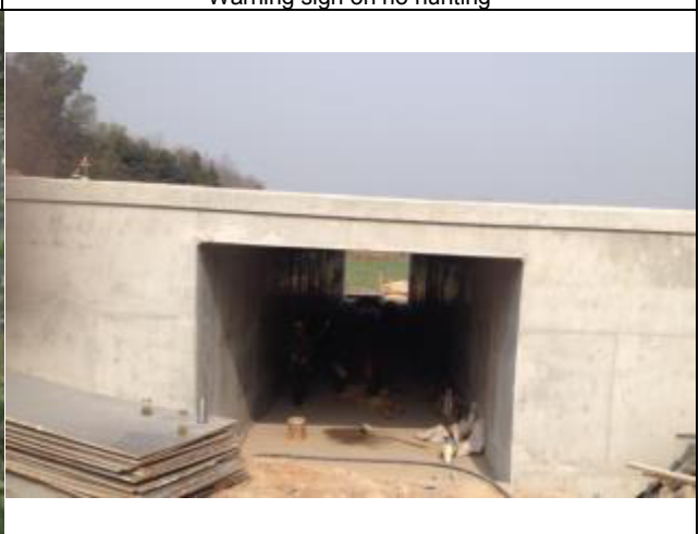
Box culvert at K0+127
