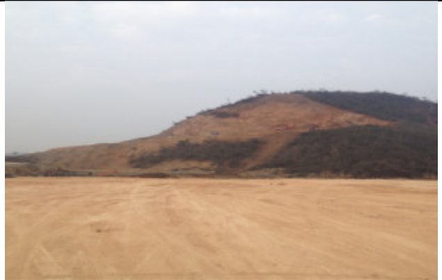
Borrow area at K14+100
