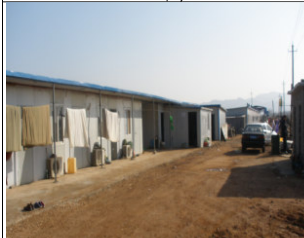
Contract NO2-1 construction camp
