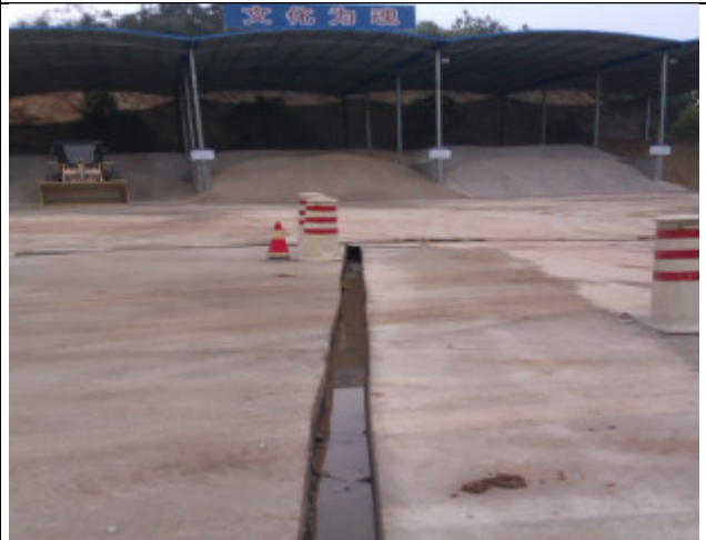
Interception ditch in asphalt mixing station
