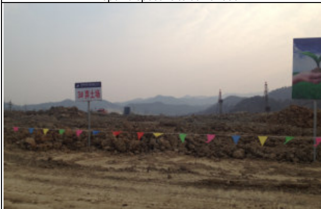
# 3 spoil disposal site at K11+120
