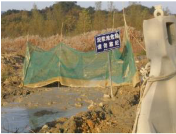
Interception ditch needed to direct process wastewater to sedimentation tank in asphalt mixing station
