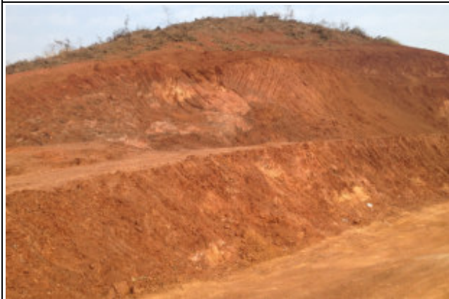
#1 borrow area at K1+500
