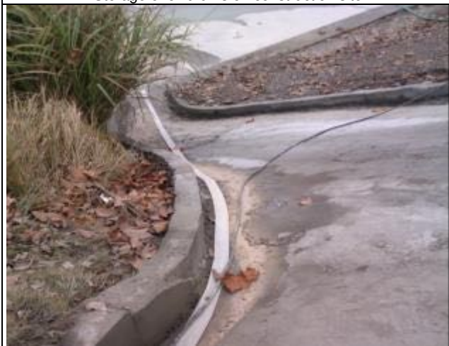
Drainage ditch in asphalt mixing station
