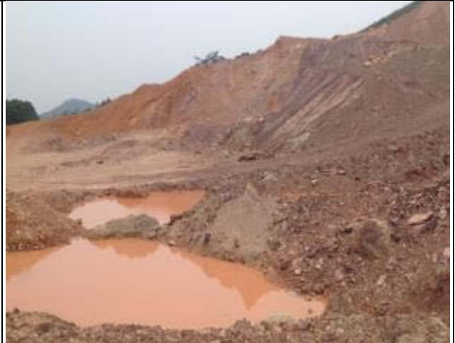
#2 borrow area with sedimentation pond to contain muddy runoff
