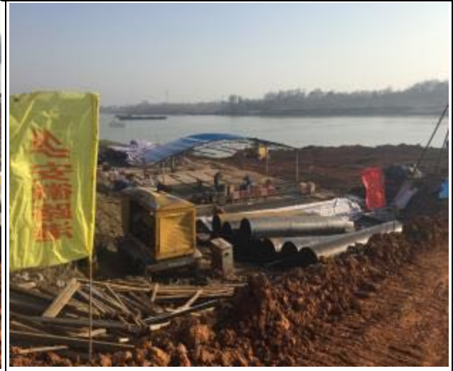
Construction site and material stockpiling
