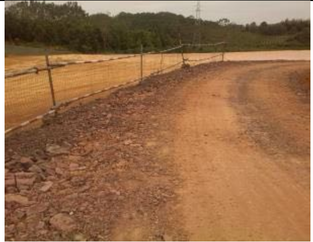
Compacted access road to reduce fugitive dust emission
