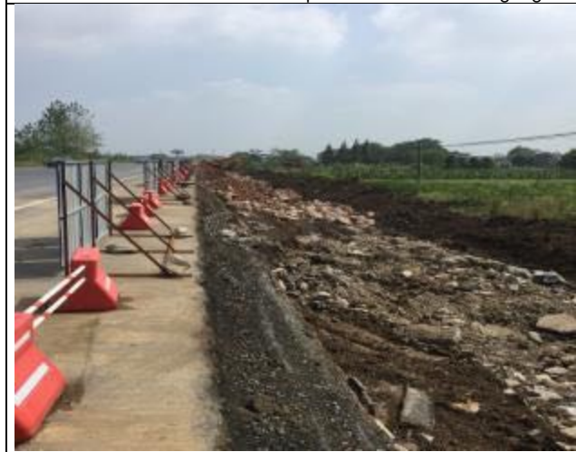
Road construction site
