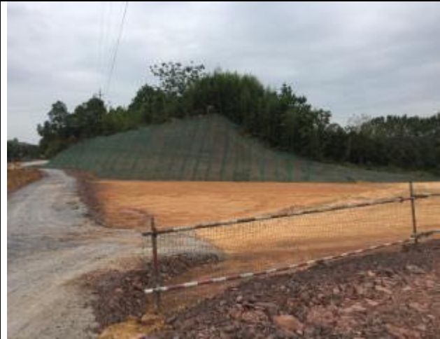
#1 borrow area with slope protection for soil erosion prevention
