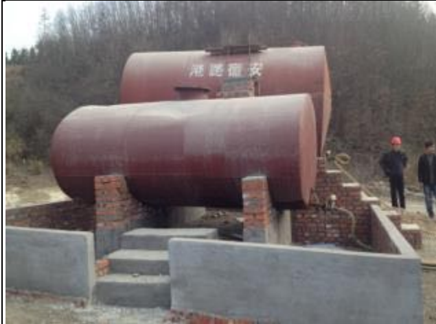
Storage of oil drums on construction site
