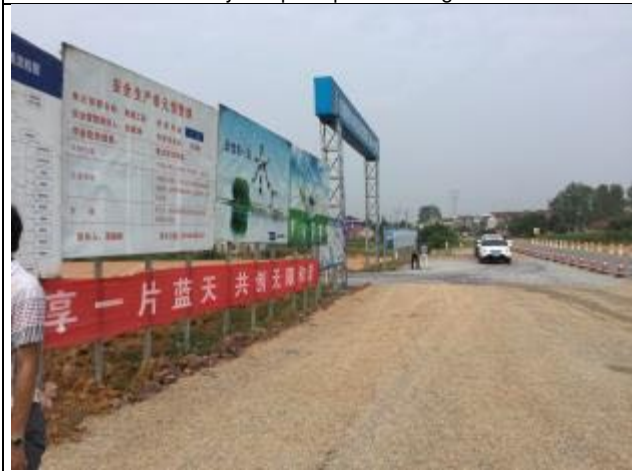
Compacted subgrade to reduce fugitive dust emission
