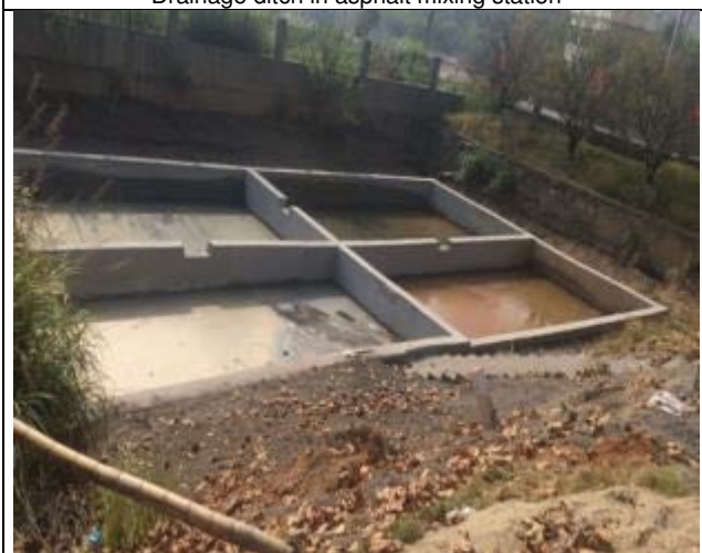
4-chamber sedimentation tank in NO2-1 asphalt mixing station
