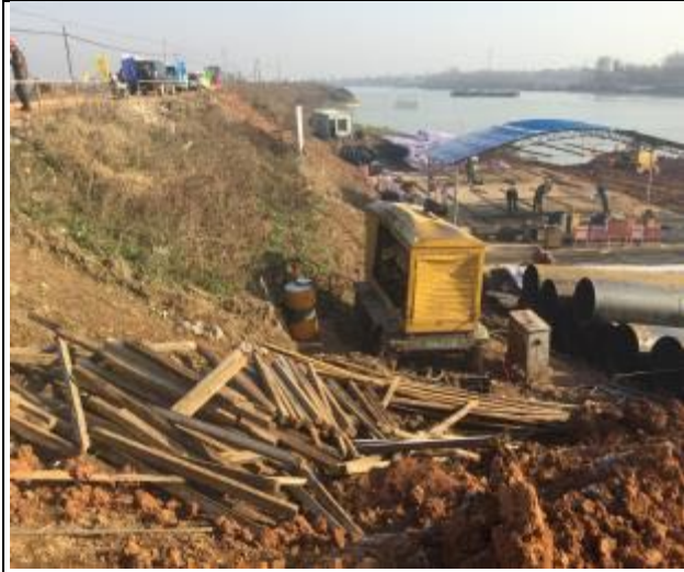
Construction material stockpiling
