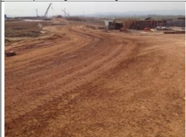
Haul road shortly after watering
