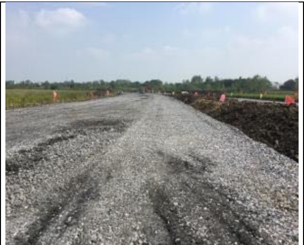
Gravel paved road for reducing fugitive dust emission from construction traffic
