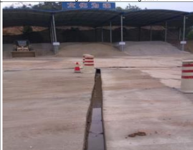
Interception ditch in asphalt mixing station
