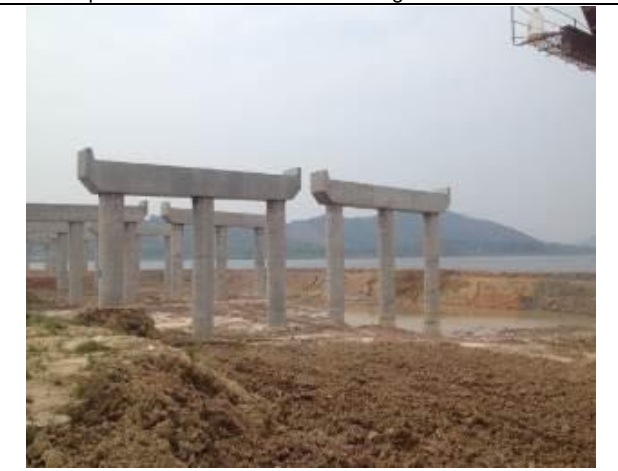
Coffer dam at Xiaohuangni Lake bridge construction site
