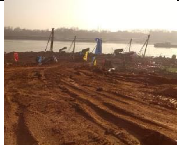
Access road to port construction site
