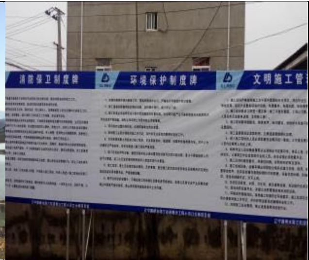
Construction site environmental protection billboard
