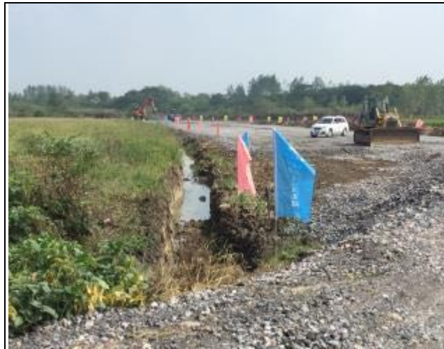
Gravel paved road for reducing fugitive dust emission from construction traffic
