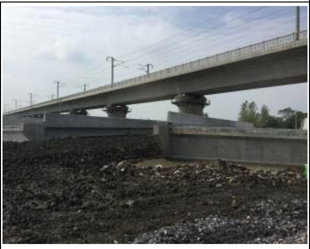
Bridge construction site
