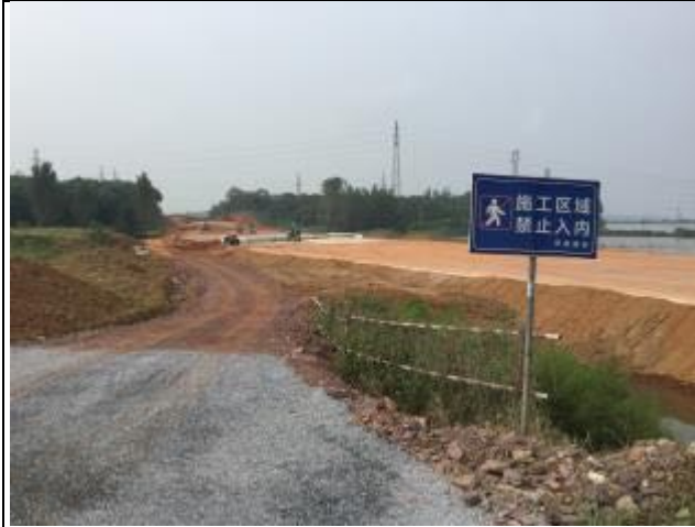
Site entry/exit point paved with gravel
