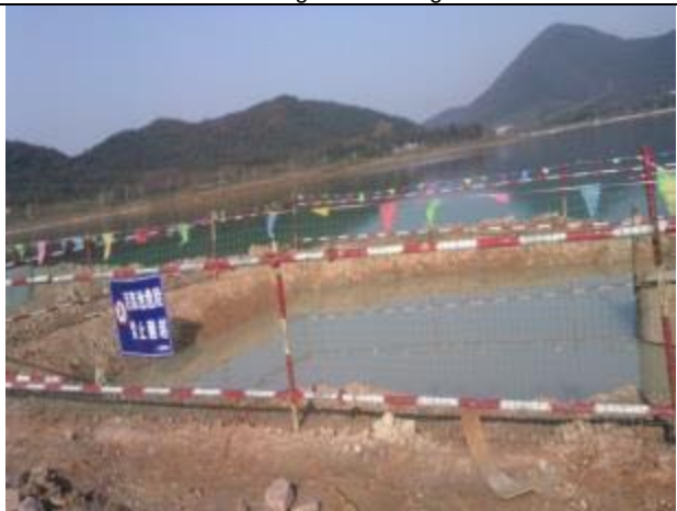
Sedimentation pond on construction site
