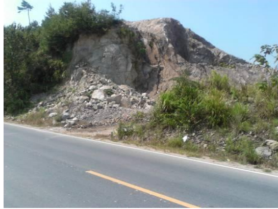
Figure2- 6 Present Situation of the Borrow Area
