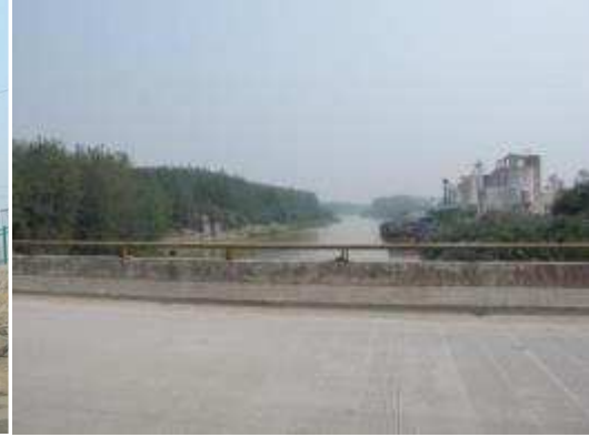
Plate III.6: Ma'anshan: Sima River Crossing
