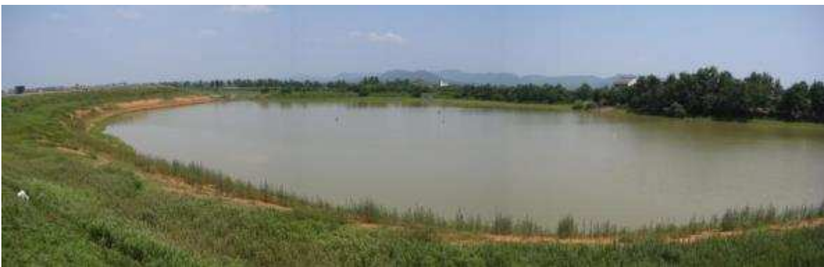
Plate III.20: Proposed dredged dumping site in pond within Shuiyang River flood bunds
