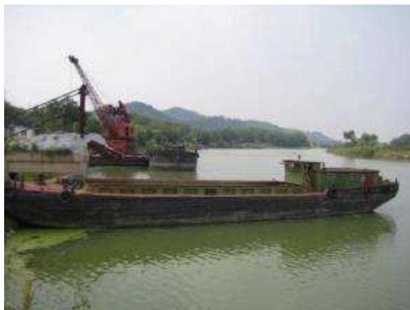
Plate III.2: Existing port on the Shuiyang River
