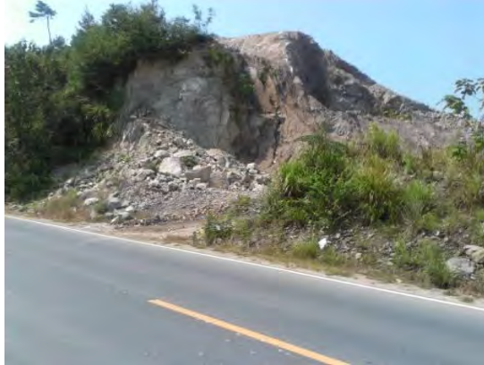
Figure 2-3 Present Situation of the Borrow Area
