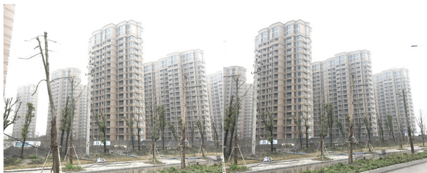
Figure 3 Resettlement houses of Chendong New District to be put in use
