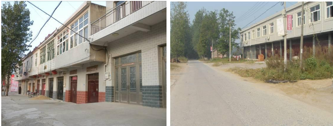
Figure 2-4 Houses beside the Segment to be Broadened
