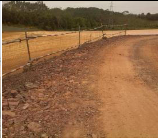
Compacted access road to reduce fugitive dust emission
