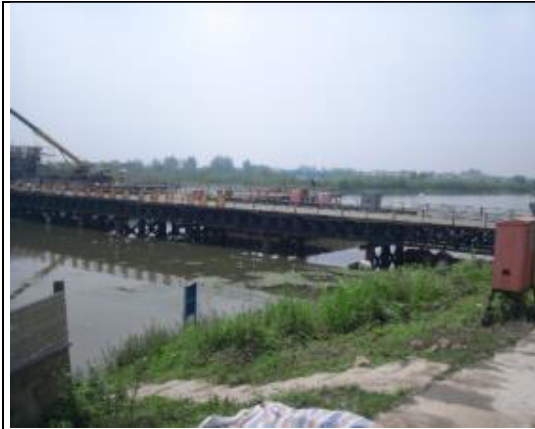
Section III bridge construction site
