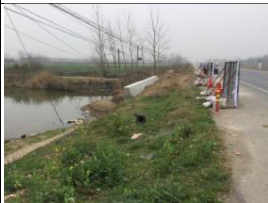
Section I road construction site
