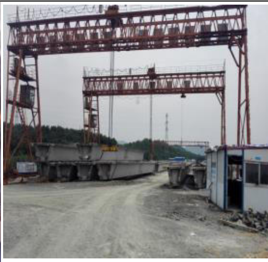
NO2-2 bridge precasting yard
