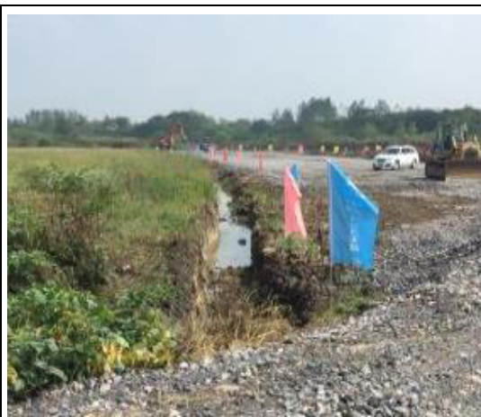
Gravel paved road for reducing fugitive dust emission from construction traffic
