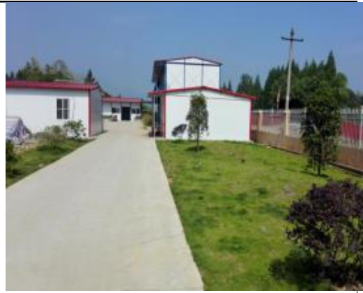
Contract NO3-1 staff dormitory
