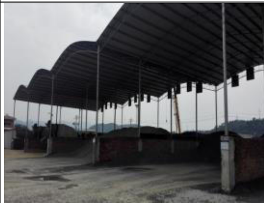
Mixing station material stockpiling
