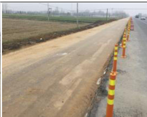
Section II road construction site
