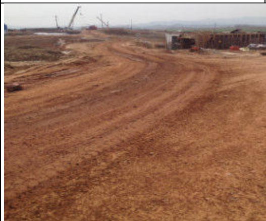
Haul road shortly after watering
