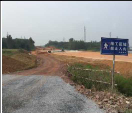
Site entry/exit point paved with gravel
