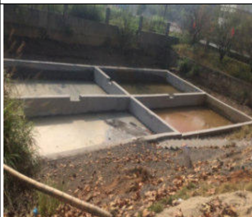
4-chamber sedimentation tank in NO2-1 asphalt mixing station
