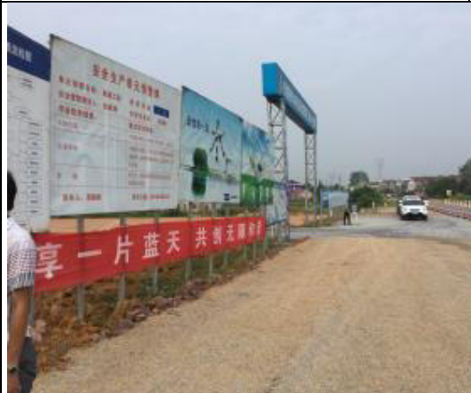
Compacted subgrade to reduce fugitive dust emission
