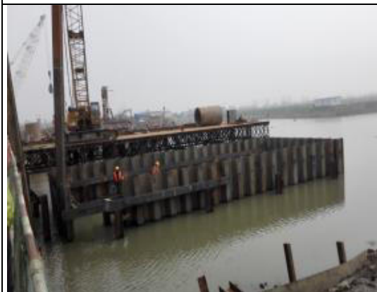
Installing steel hoardings to protect water bodies in bridge construction
