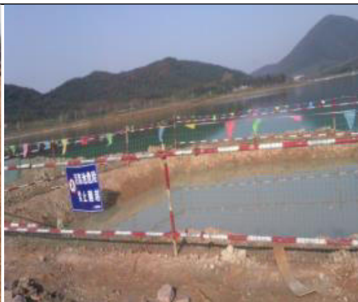
Sedimentation pond on construction site
