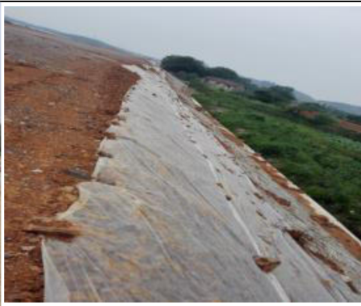
Road subgrade side slope for soil erosion prevention
