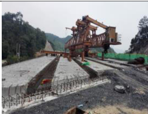
Meigong Bridge construction site
