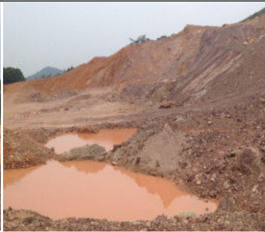
#2 borrow area with sedimentation pond to contain muddy runoff
