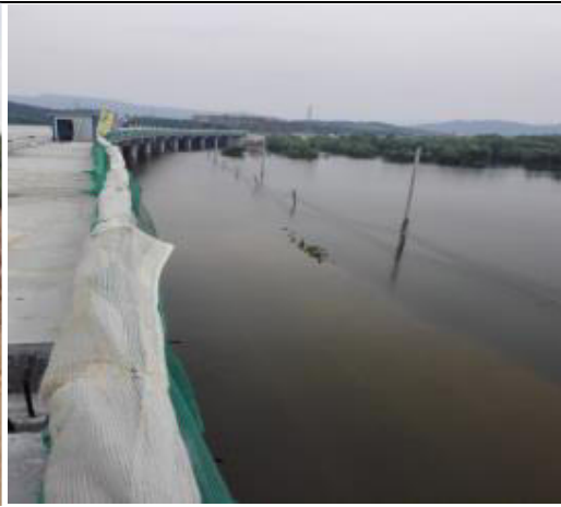
Xiaohuangni Lake construction site
