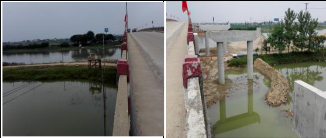
Construction sites near Xiaohoukou bridge location
