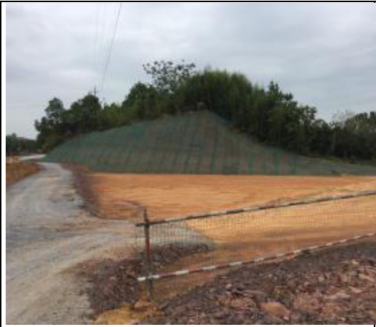
#1 borrow area with slope protection for soil erosion prevention
