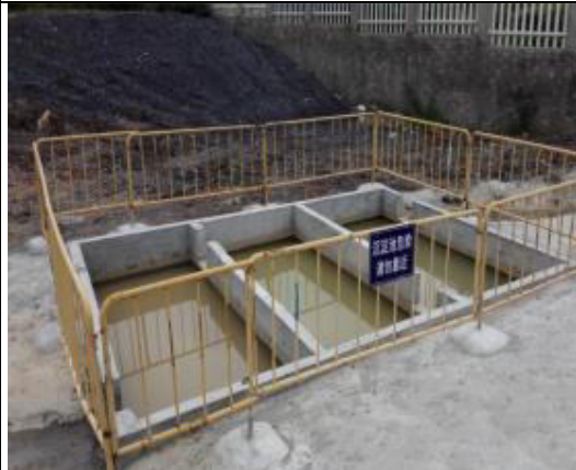
Sedimentation pond at mixing station
