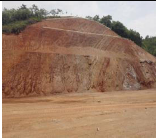
Stair-shaped borrowing in borrow area
