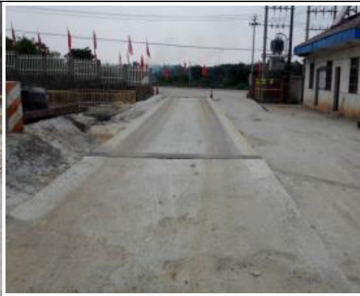
Access road to construction site at mixing station
