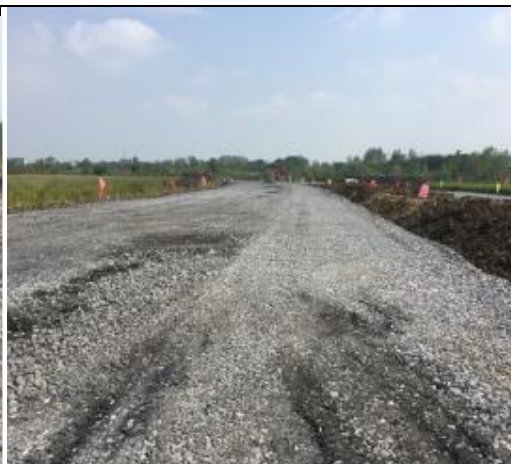
Gravel paved road for reducing fugitive dust emission from construction traffic
