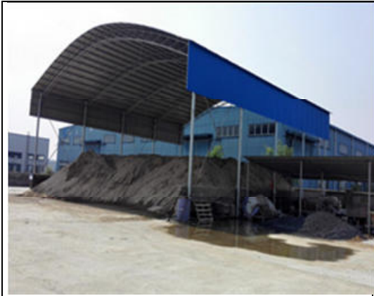
Contract NO3-2 mixing station
