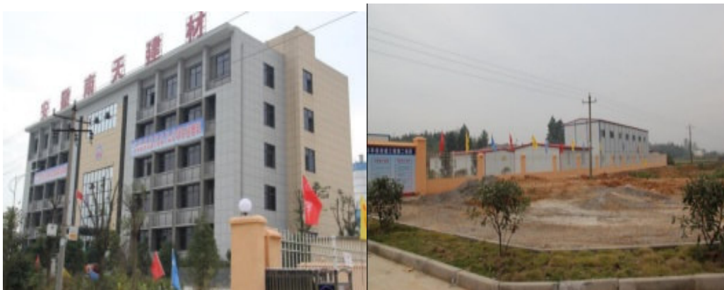
Picture 10 Residential office and rented yard in Contract No.02
