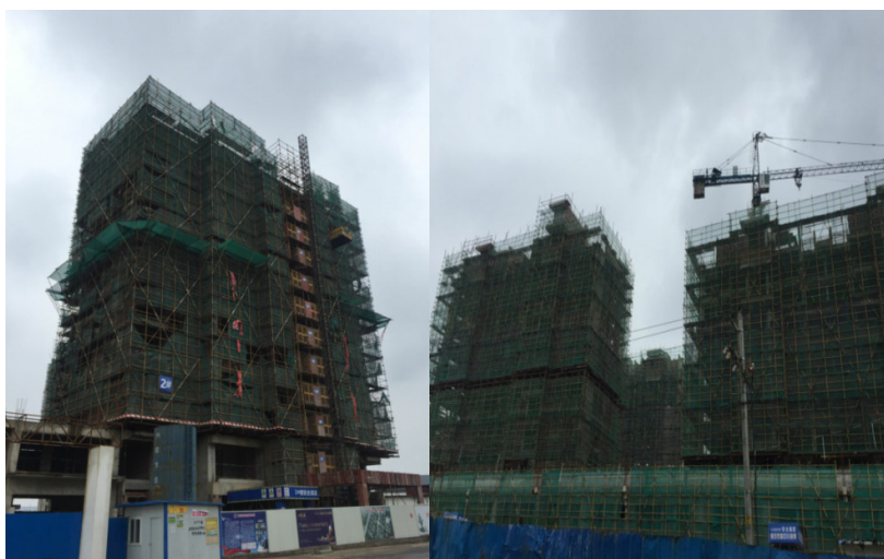
Picture 6 Huishang Century City Settlement
