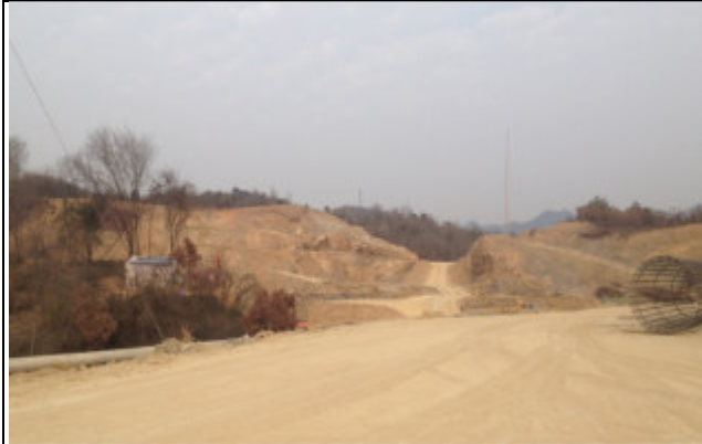
Borrow area across from the site office
