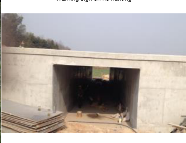
Box culvert at K0+127
