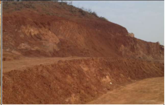
Terraced soil excavation to minimize soil erosion
