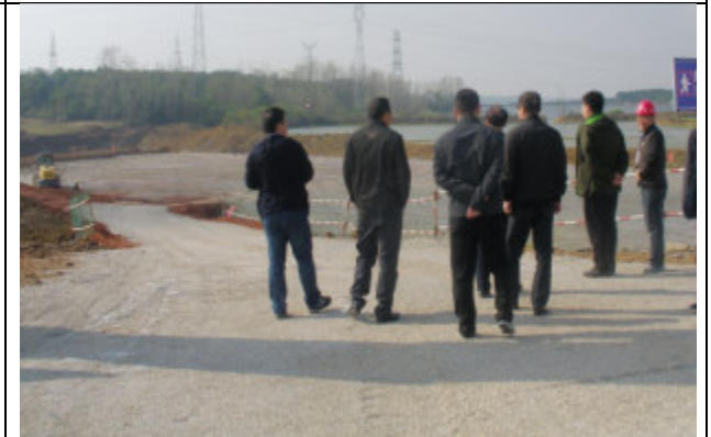
Access road at K13+800 paved with gravel to minimize fugitive dust emission
