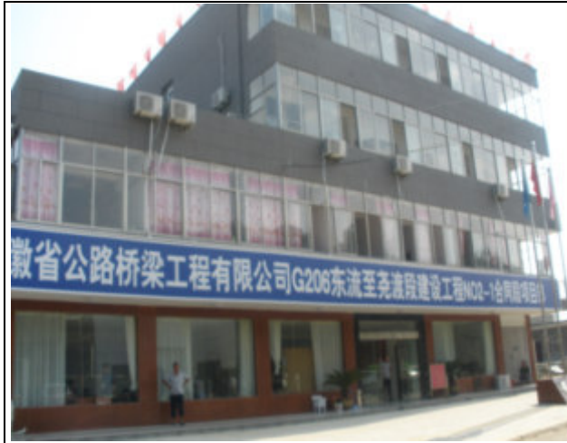
Contract NO2-1 project office
