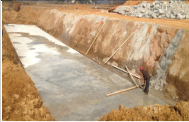
Cement sprayed on culvert sides to minimize soil erosion
