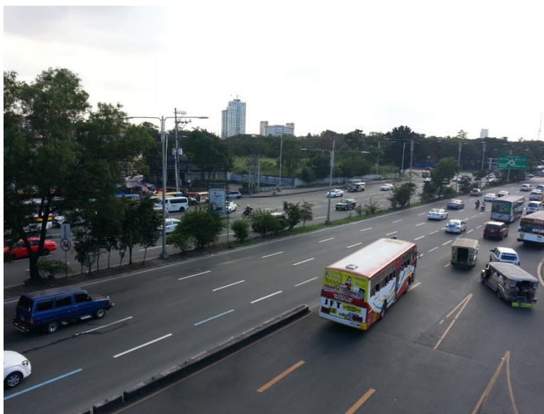
Commonwealth Avenue, viewed on its approach to Elliptical Road
