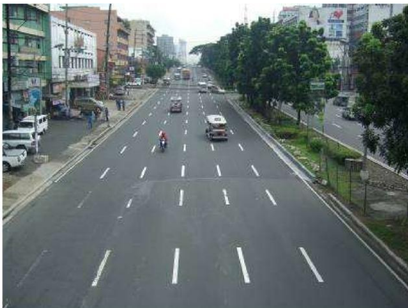
Quezon Avenue, on approach to Araneta intersection
