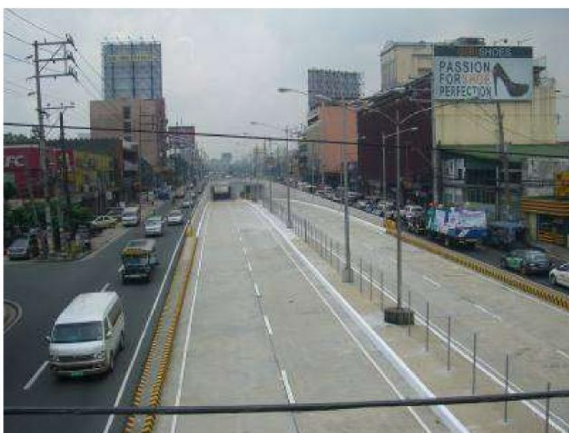
Quezon Avenue, looking towards the recently constructed Araneta Underpass
