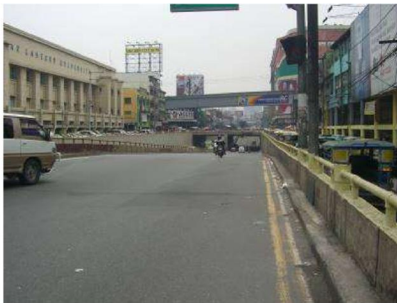
España Boulevard, looking towards underpass and Recto Avenue
