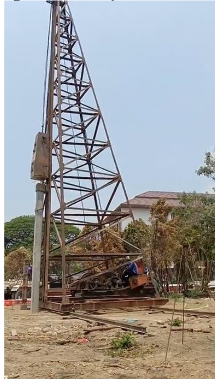
Figure 14: Example of Pile Frame
