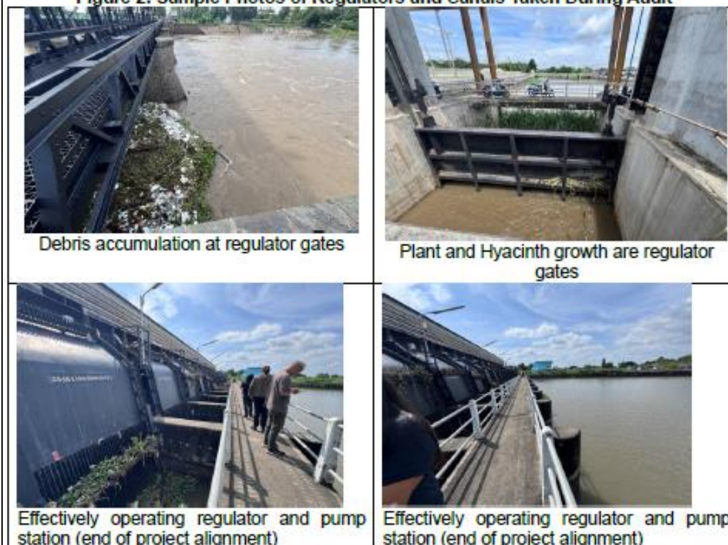
Figure 2: Sample Photos of Regulators and Canals Taken During Audit
