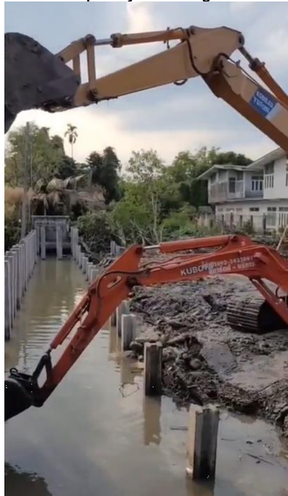
Figure 13: Example Layout of King and Batter Piles
