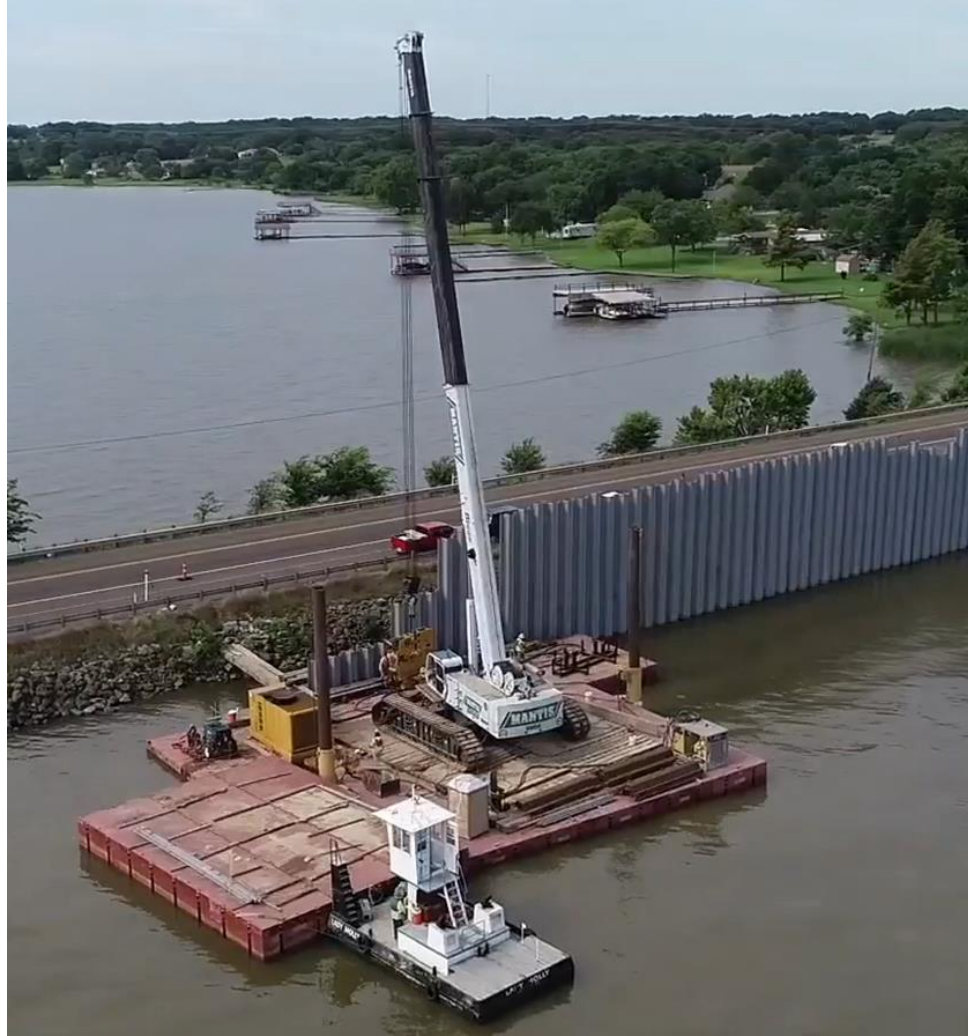
Figure 15: Example of Piling from Barge
