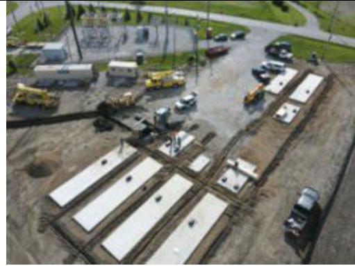
Battery pad construction
