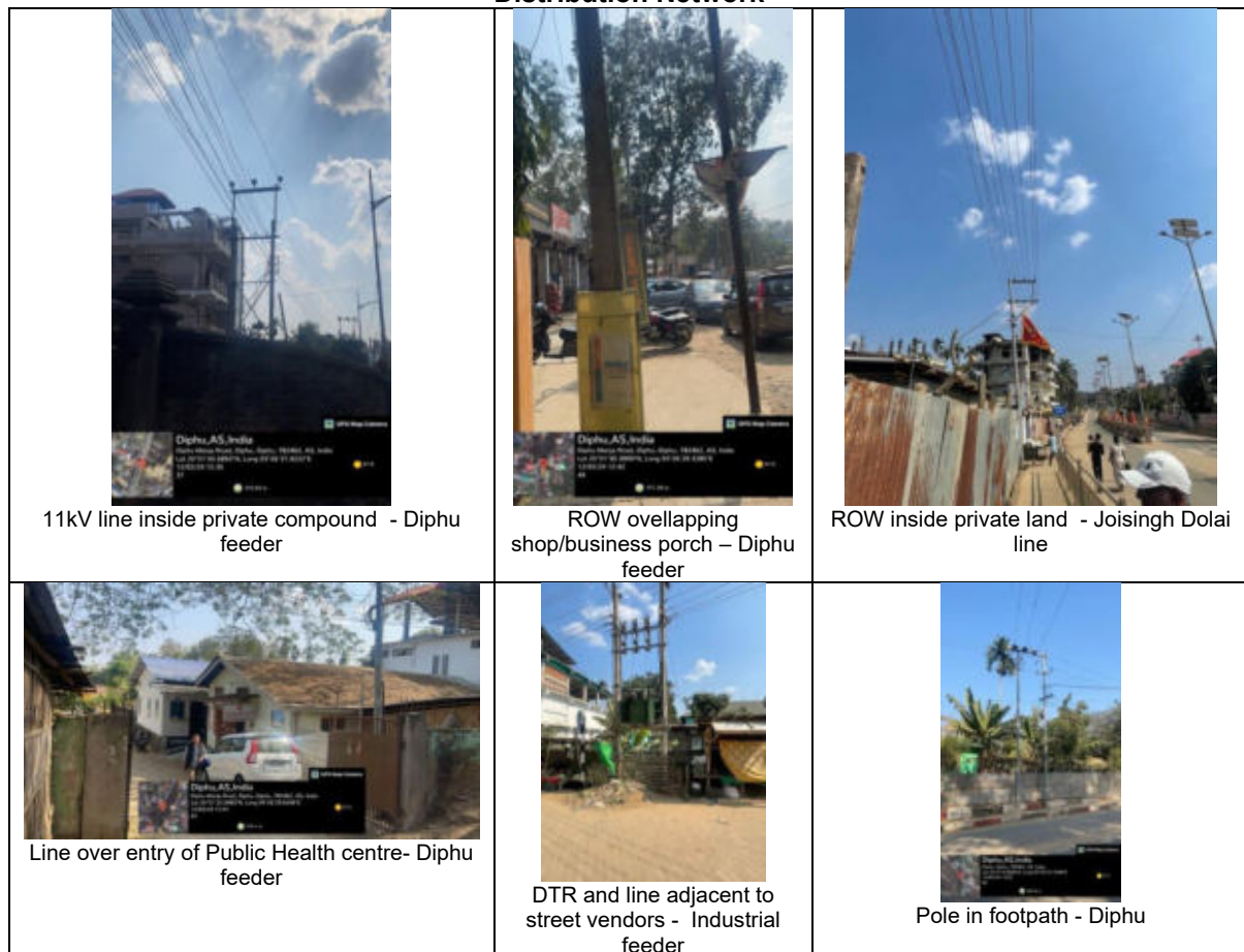
Figure 5.8 Community H&S Risks Associated with Distribution Line ROW and Operation of Distribution Network
