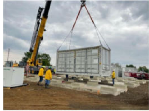
Battery module installation
