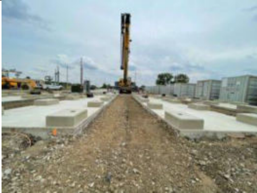
Completed battery pads
