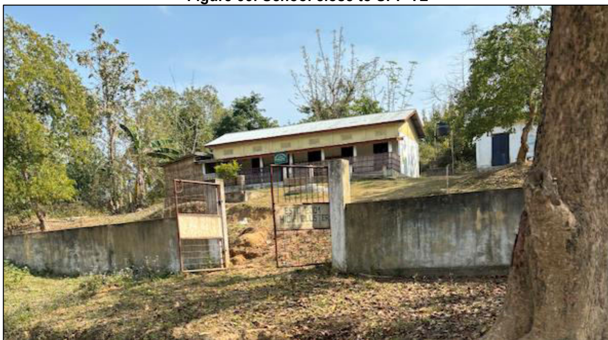
Figure 66: School close to SPP TL
