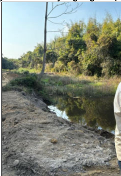
Figure 37: Recently dug irrigation pond
