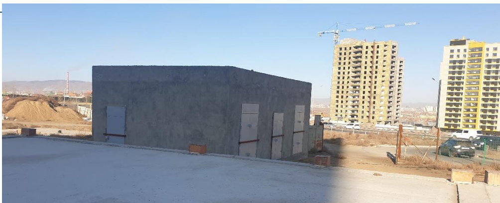
Figure 5-2. The Rower Substation
