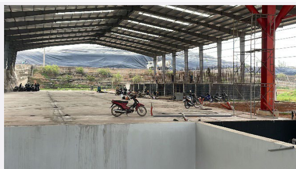
Photo 17: Compost plant under construction. Civil engineering works for waste reception hall and picking line.
