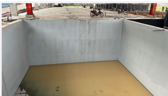
Photo 31: No fall barriers in place around the waste reception area of the new compost plant; estimated 5-7m drop.
