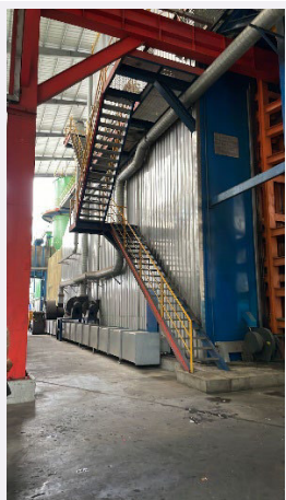
Photo 3: Incinerator chamber.
