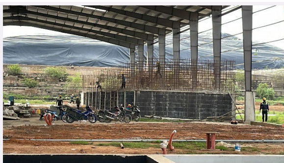
Photo 32: Third party contractor undertaking form work and concrete pour for dirty material recovery facility at new compost plant without fall protection measures.
