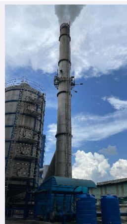
Photo 8: Stack for 8,400 kg/hour WtE.
