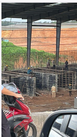
Photo 33: 3 rd party contractor undertaking form work and concrete pour for dirty material recovery facility at new compost plant without fall protection measures.
