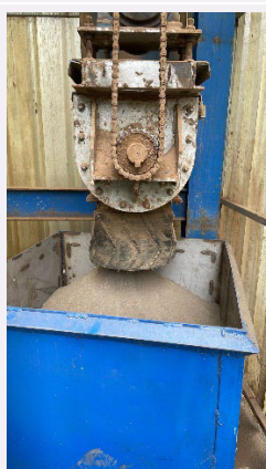
Photo 9: Close-up photo of a fly ash hopper.
