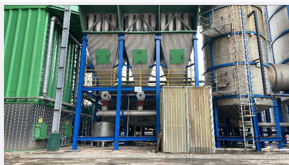
Photo 5: Fly ash hoppers, ash is also sent to the brick manufacturing plant.
