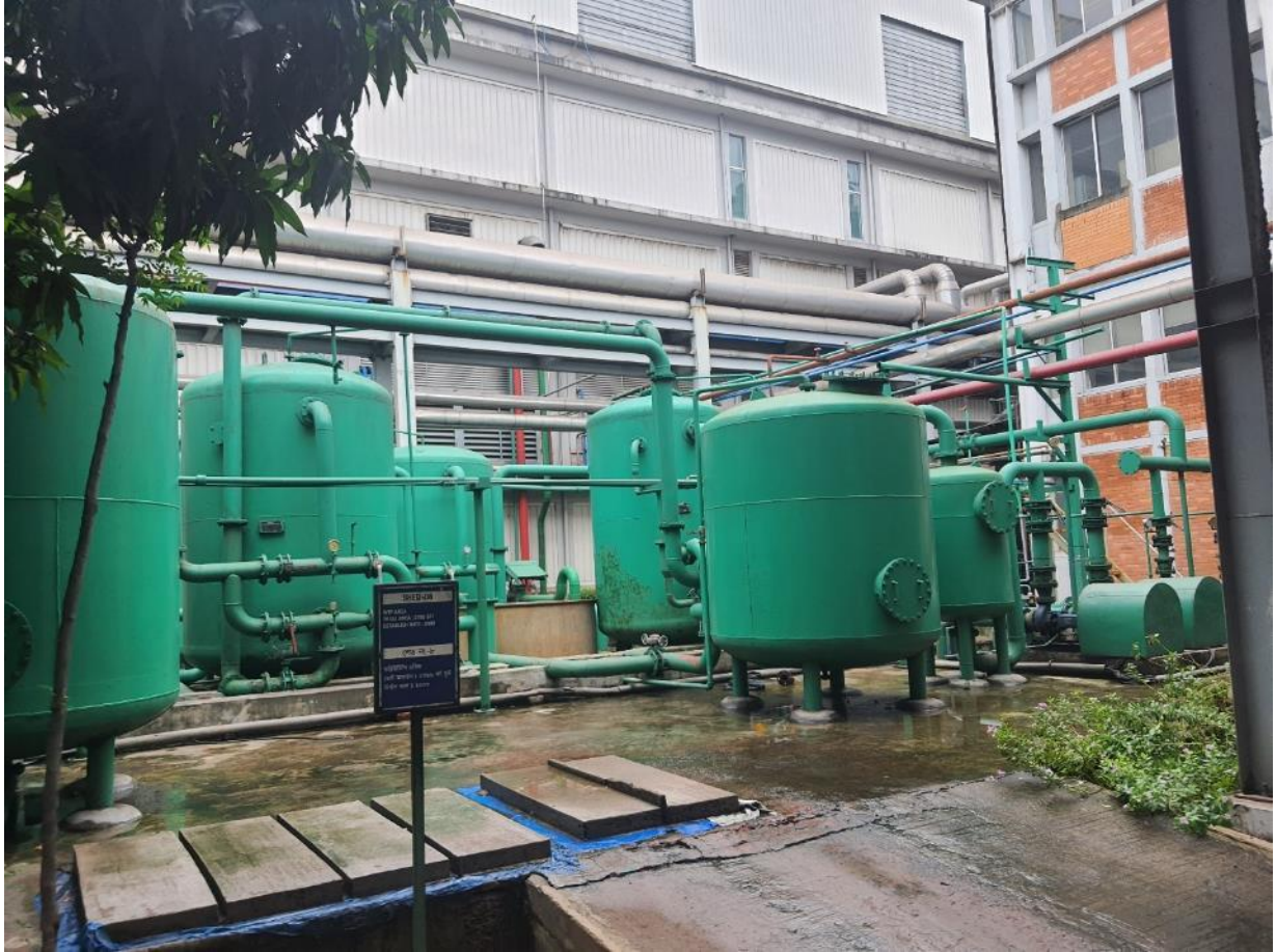
Figure 20 Effluent Treatment Plant (ETP)
