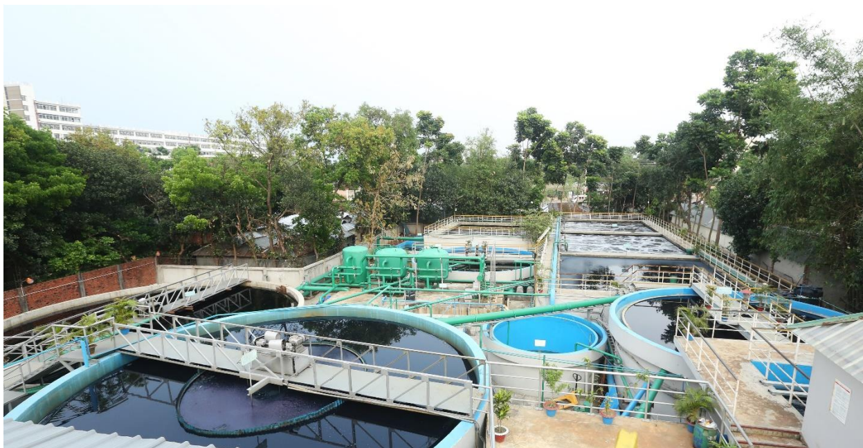
Figure 5 Effluent Treatment Plant of ETL
