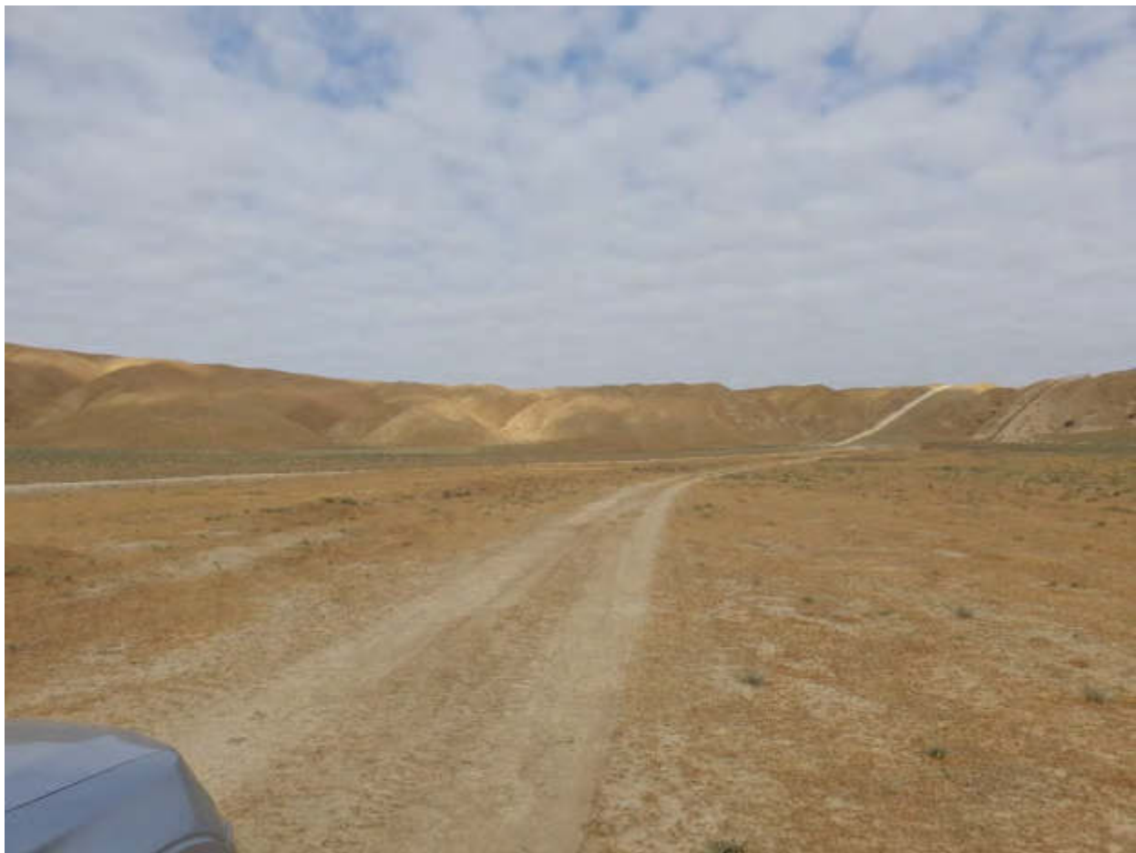
Figure 1-2: Example section of the existing track to be used for the new access road
