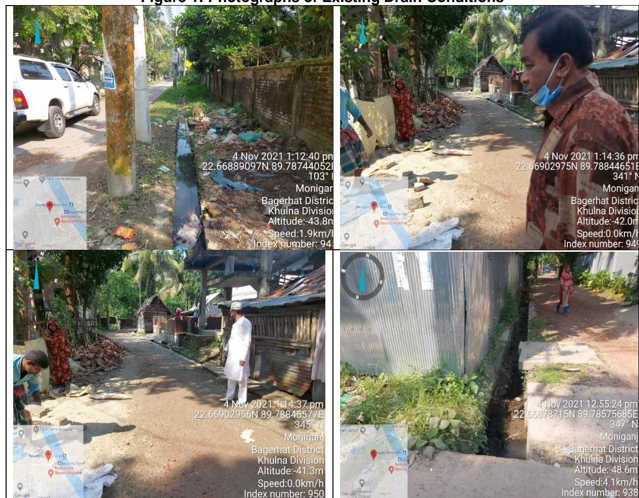
Figure 1: Photographs of Existing Drain Conditions
