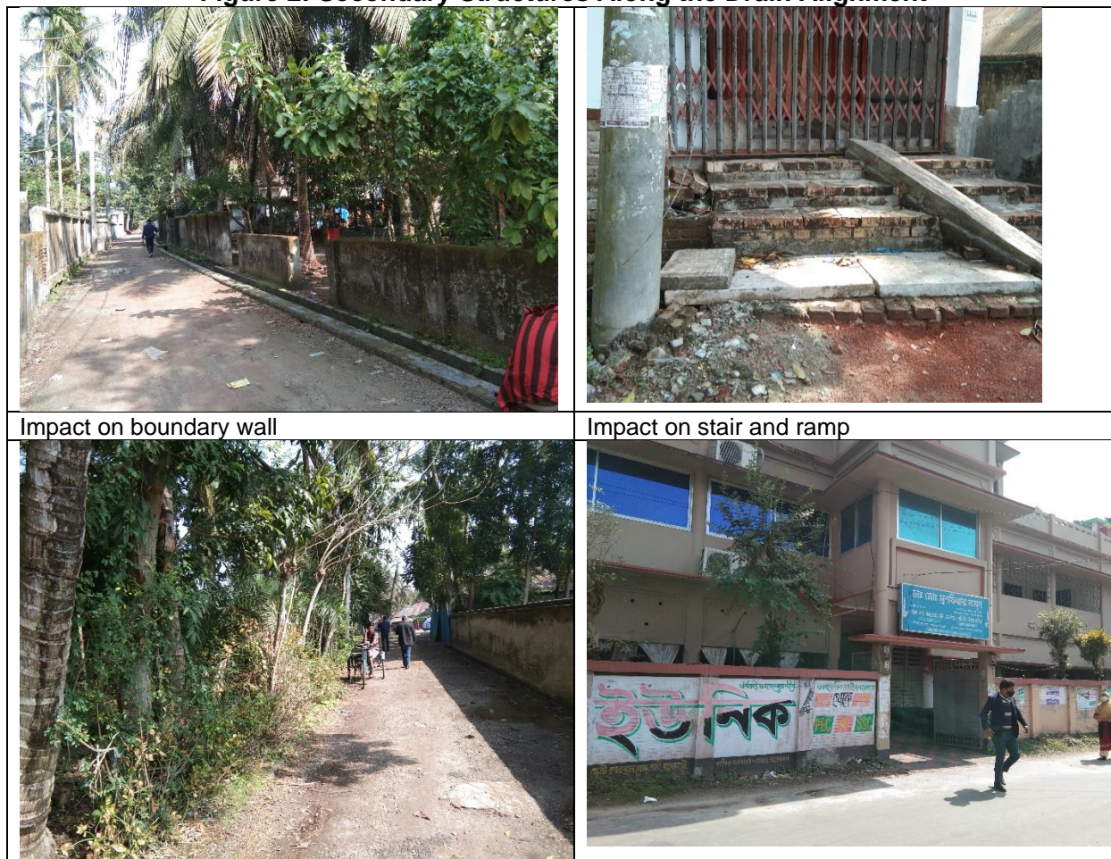
Figure 2: Secondary Structures Along the Drain Alignment
