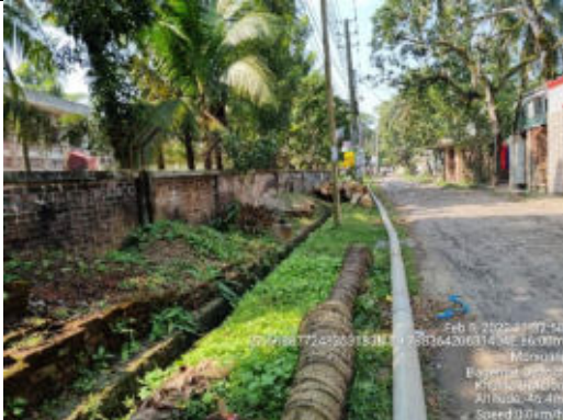
Poor condition of existing drain
