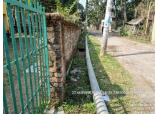
Widening or repairing will affect school boundary wall
