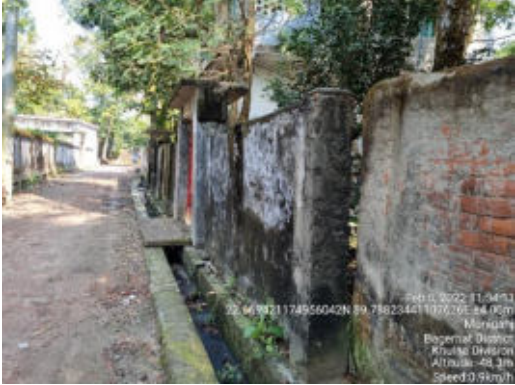
Boundary wall that might be affected
