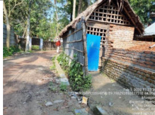
Private land over encroched into the drain
