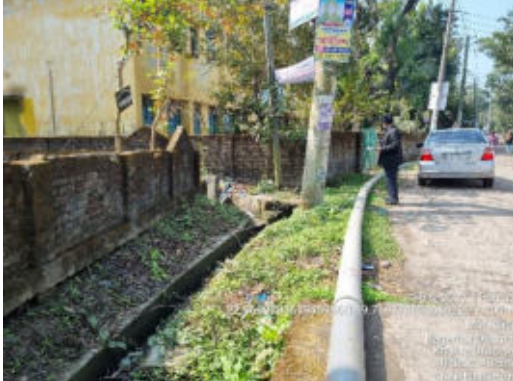
Widening or repairing will affect boundary wall
