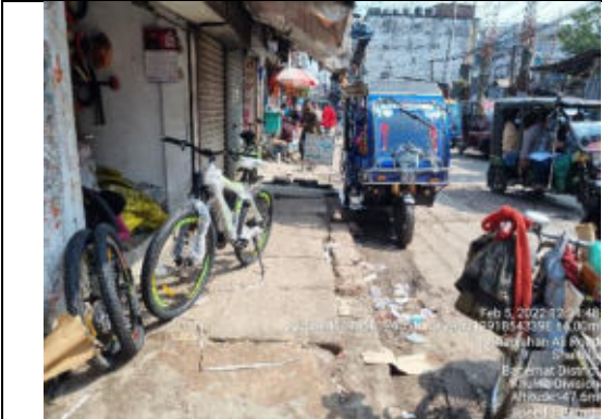
Drainage canal alignment in the busiest area of Bagerhat municipality
