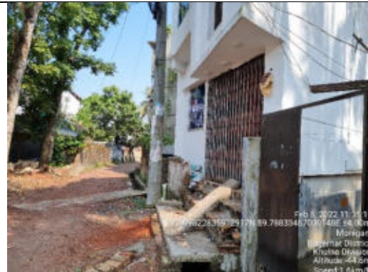
Newly build house and its ramp might be affected
