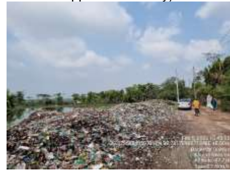
Access road of the land filling site
