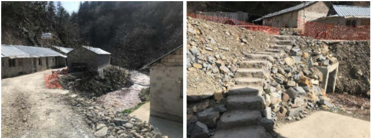
Figure 5.46: Unsafe stairs with no handrail in Zvare accommodation camp
