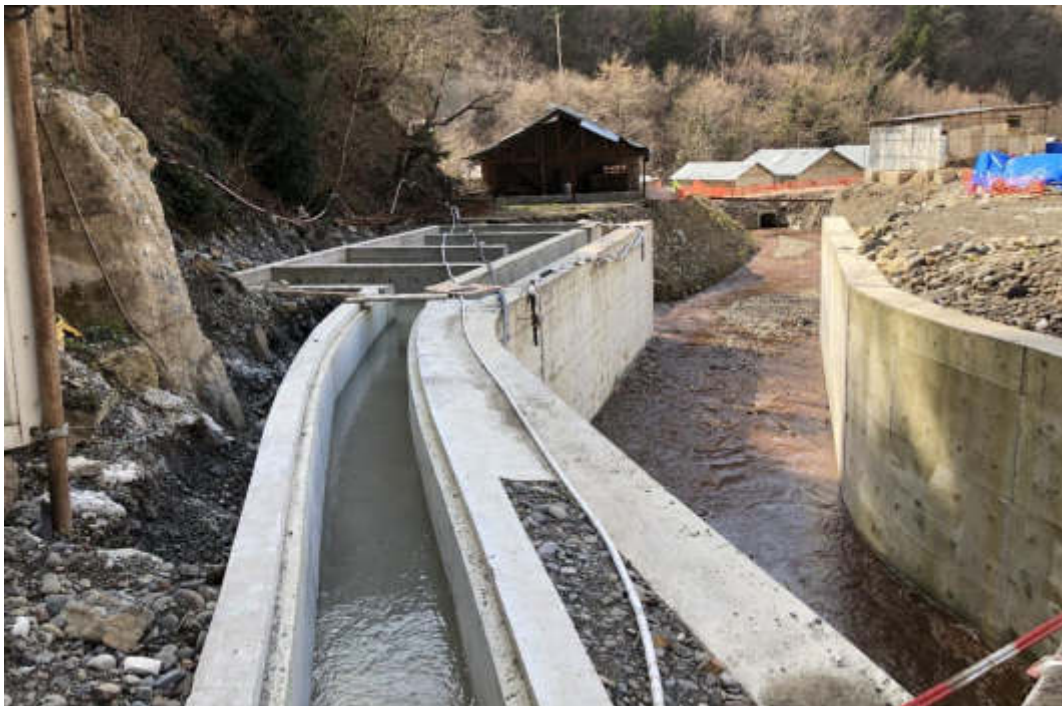
Figure 5.33: Settlement reservoir for drainage water from the Tunnel#9
