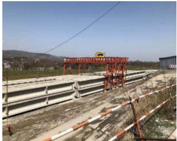
4) Bridge beams prepared for transportation
