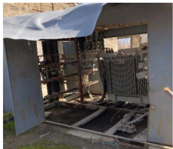
Figure 5.28: Power substation in Kvishkheti camp
