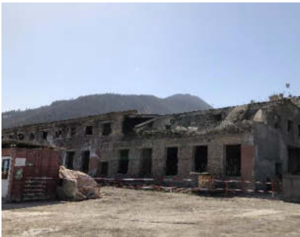
Figure 5.16: Unsafe old buildings in Kvishkheti camp
