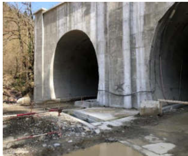
2) Tunnel #9 western portal
