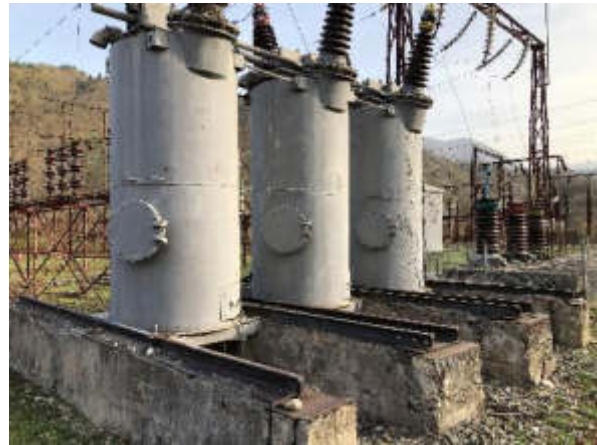
Figure 5.32: PCB-containing oil in high-voltage switches of the old Moliti power substation
