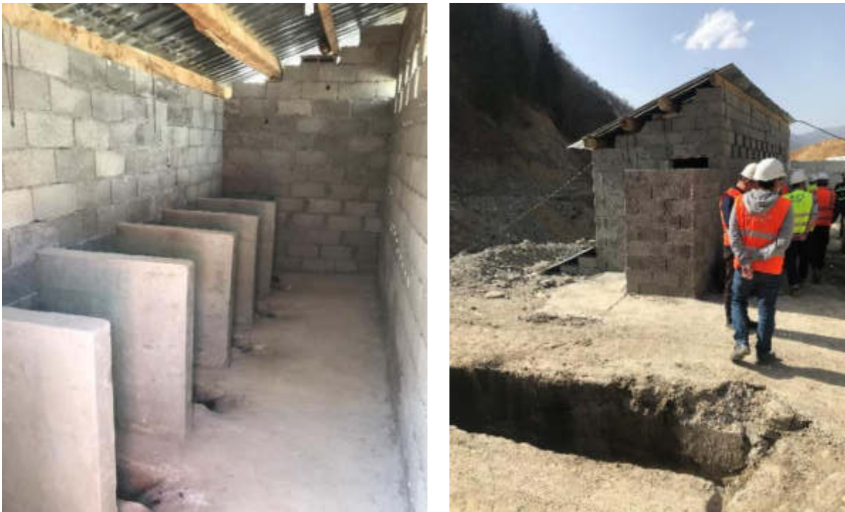
Figure 5.43: Toilet and the way to the toilet with a pit (not barriered) in Zvare camp
