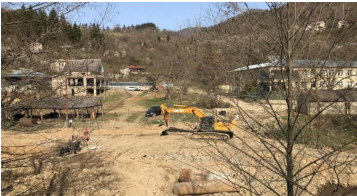
Figure 5.48: Construction site (not properly fenced), school and residential houses in Zvare
