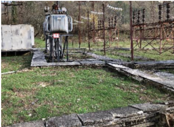
Figure 5.31: Asbestos slabs covering the cable channels at the old Moliti substation
