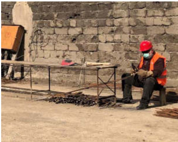
Figure 5.27: Welding in sunglasses/ face shield off
