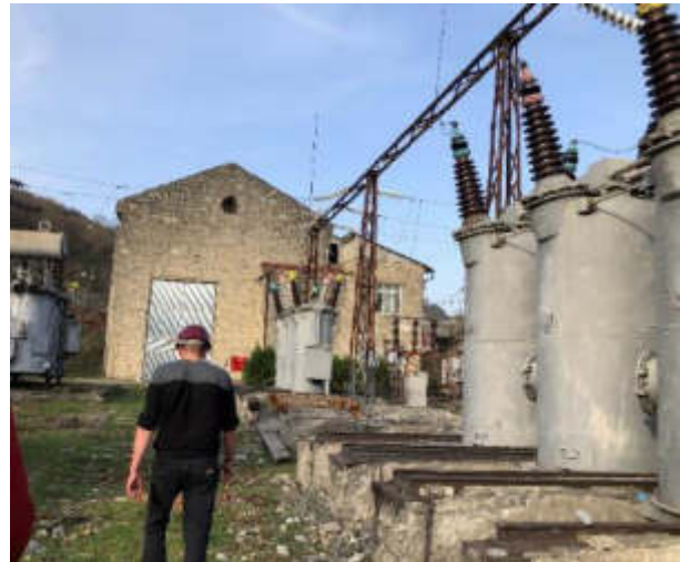
Figure 5.12: Old Moliti power substation
