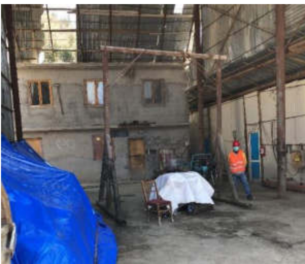
3) Machinery repair box
