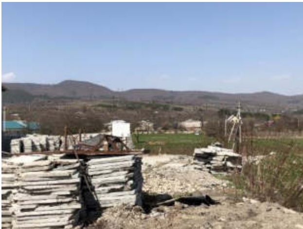
Figure 5.18: Damaged / improper fencing in Kvishkheti camp
