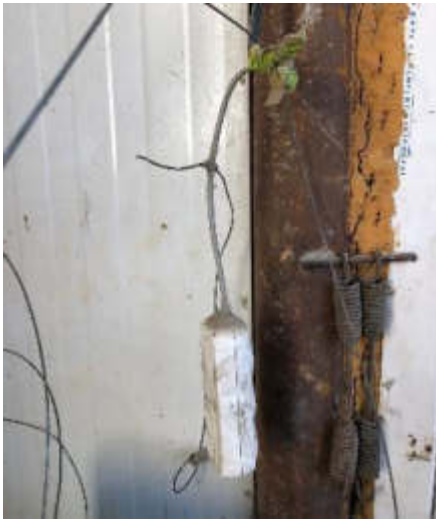
Figure 5.22: Damaged household-type extension cords
