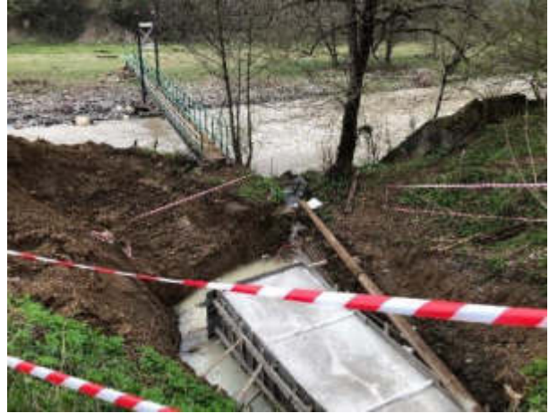
Figure 5.8: Culvert construction in Lashe Village
