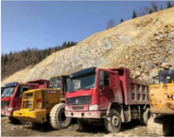
5) Construction machinery parking
