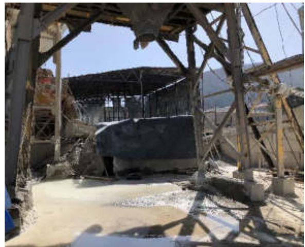
Figure 5.17: Condition of the batching plant structures in Kvishkheti
