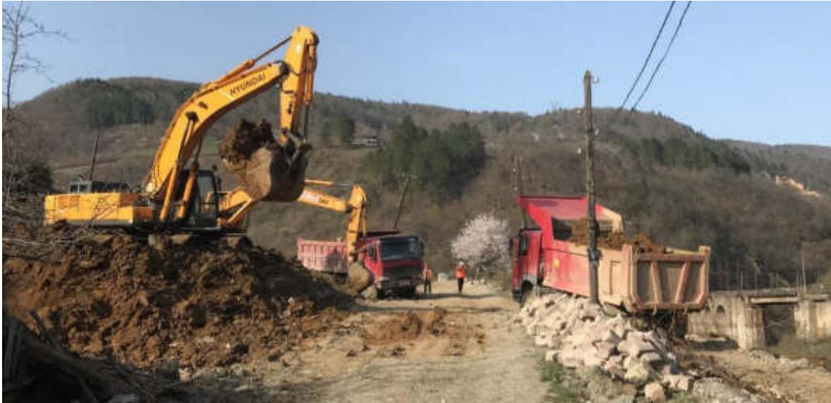
Figure 5.49: Construction site in Aneula
