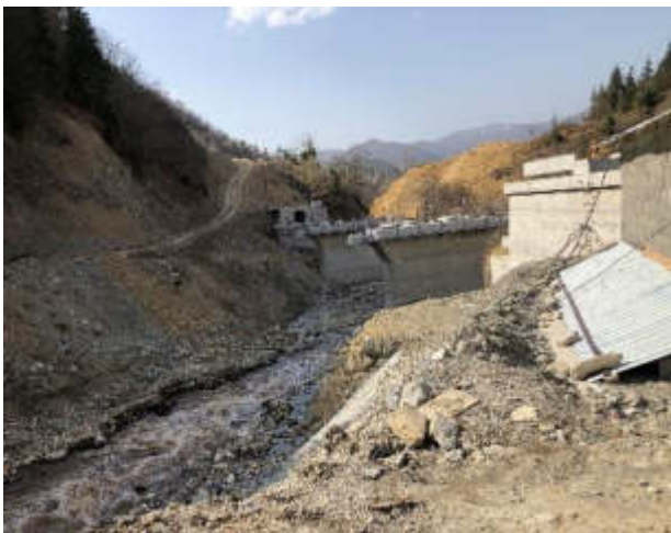
Figure 5.5: Bridge construction in Zvare camp
