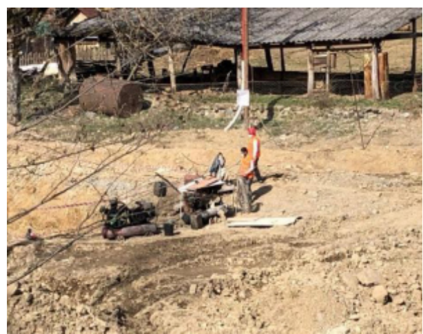
Figure 5.6: Piling works in Zvare Village.
