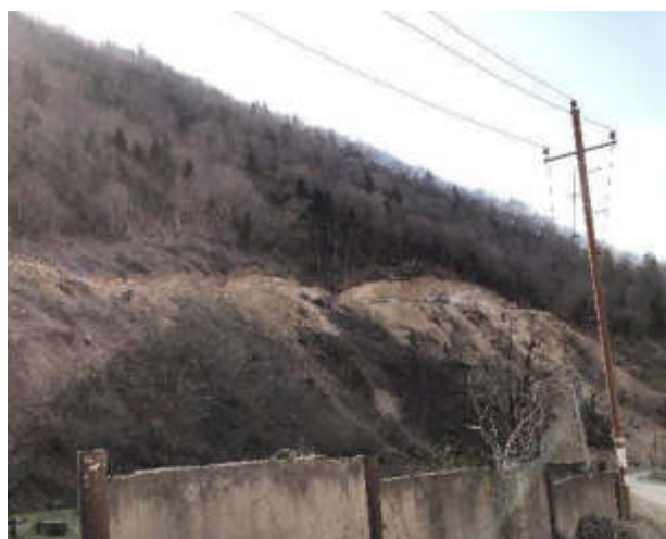
Figure 5.10: Wood cutting near Zvare
