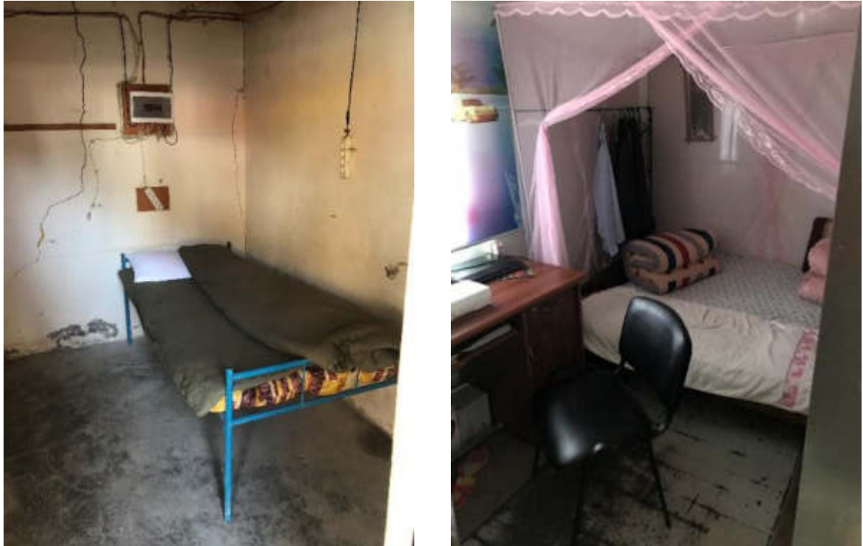
Figure 5.45: First Aid Rooms in accommodation camps in Zvare (left) and Bazaleti (right)
