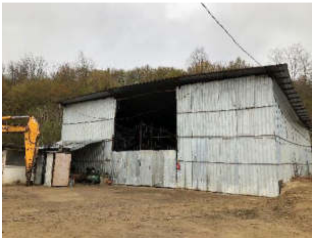
1) Warehouse/ metal workshop
