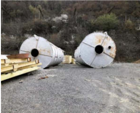
1) Dismantled batching plant area
