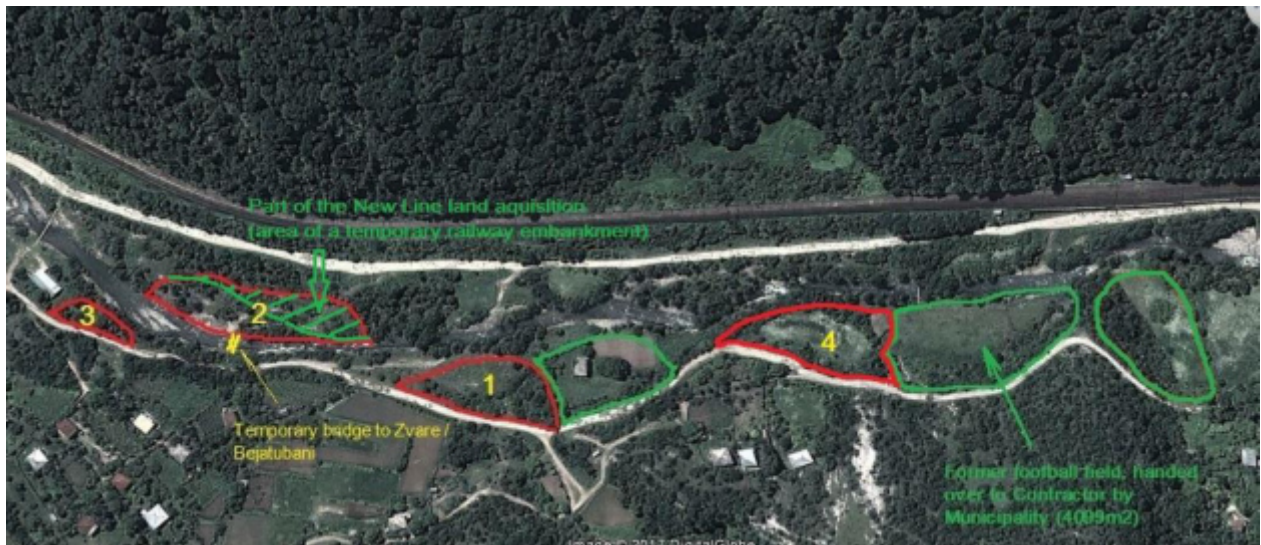
Figure 5.36: Legal and illegal spoil grounds near Aneula Village in March 2019 (Source – ILF Consulting, March 12, 2019)
