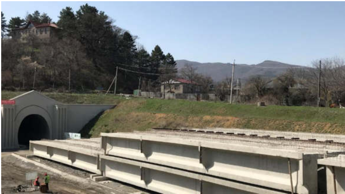
Figure 5.50: The entrance to Tunnel #9 in Kvishkheti, nearby residential houses and cattle
