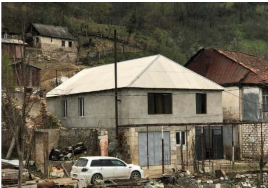
Figure 5.52: The new house of a resettled family in Dzirula (construction works are in process)
