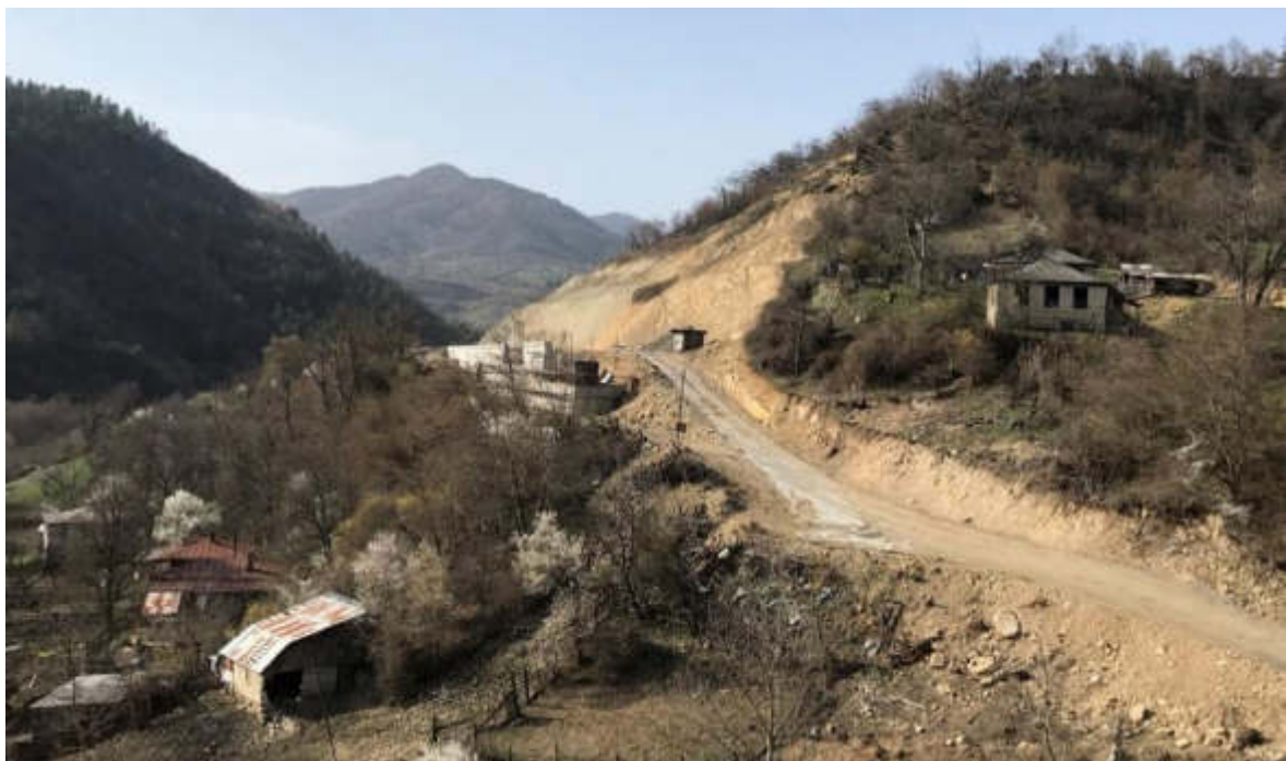
Figure 5.51: The area of the future bridge in Zvare and nearby residential houses
