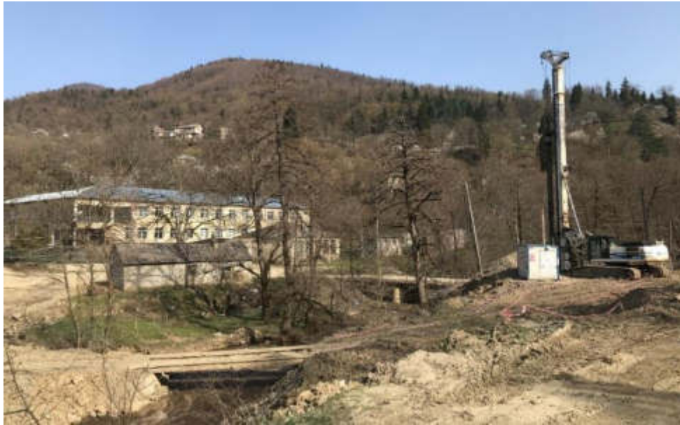
Figure 5.47: Construction site and school in Zvare
