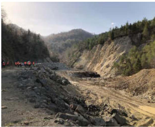
Figure 5.9: Waste rock dump near Zvare
