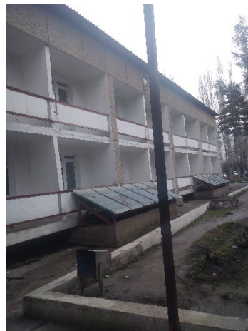
Asbestos contained roof materials
