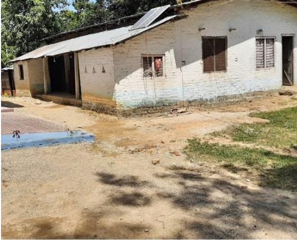
Photo 11: An old building need to be removed from construction site in Bhediya APO
