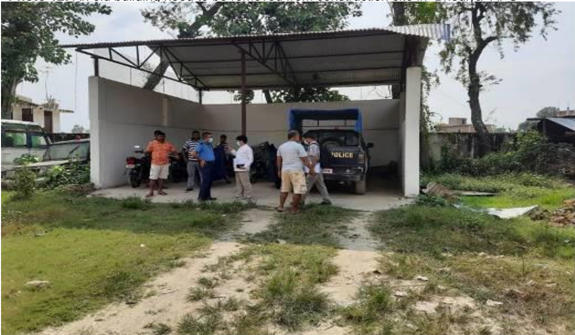
Photo 13: A Car garage need to be relocated from construction site of Gaushala APO
