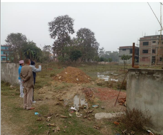
Photo 9: WCSCSC construction location of DPO Rupandehi
