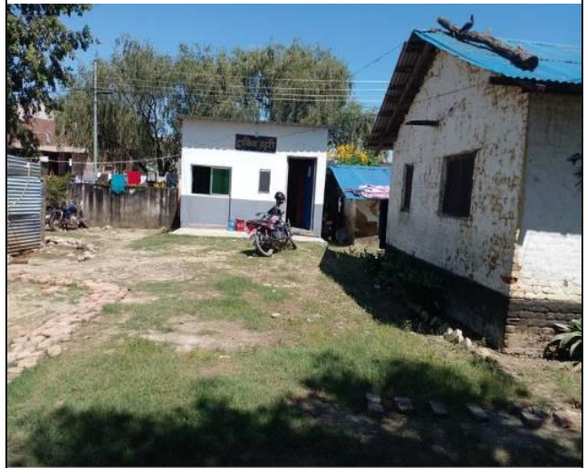
Photo 10: One roomed Traffic post to be relocated and unused old barrack& toilet are to be demolished at WCSCSC location of Tikapur
