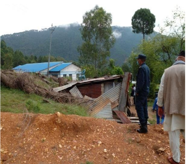
Photo no. 7: Electric pole and kitchen hut to be demolished at WCSCSC location of Patan
