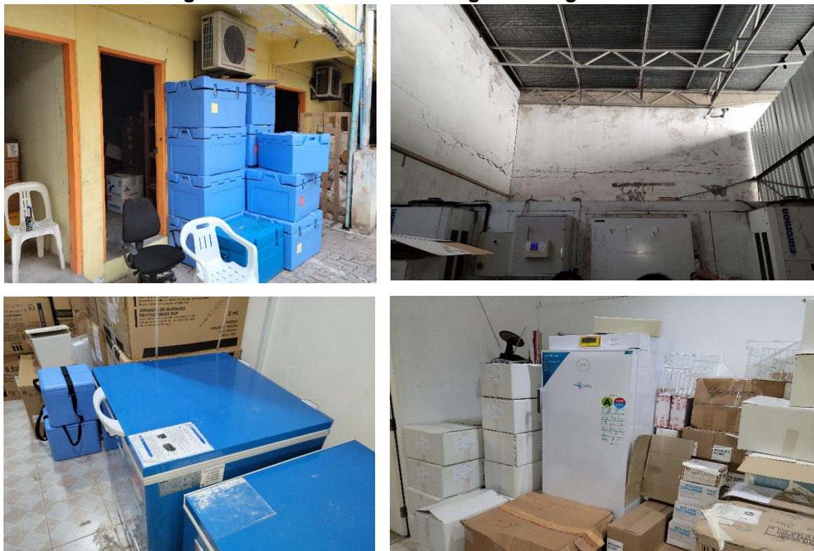
Figure 1: Central Vaccine storage building in Male'
