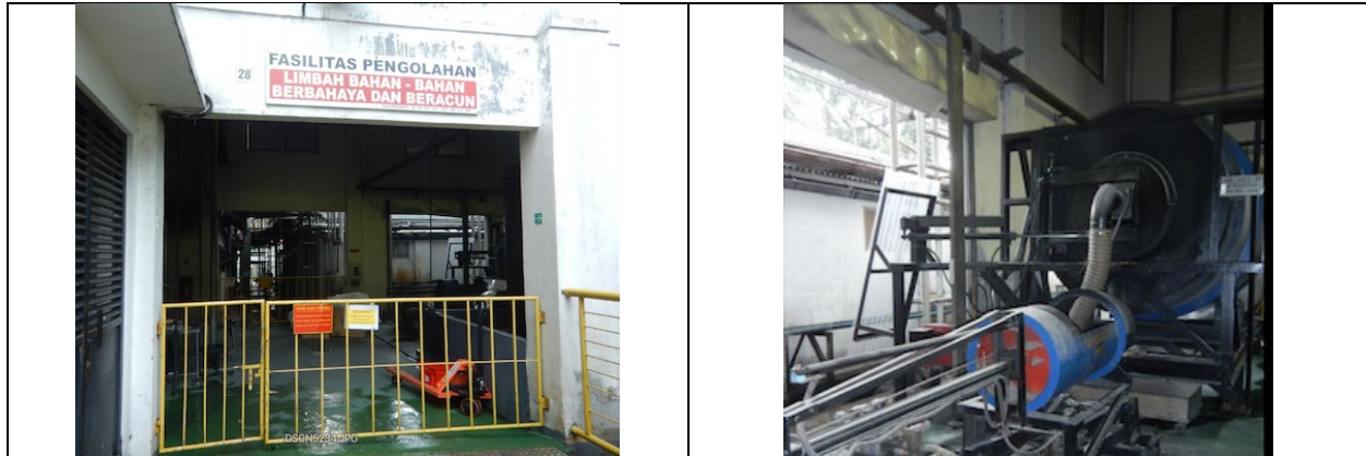
Figure 30: Existing incinerator at Bio Farma Pasteur site
