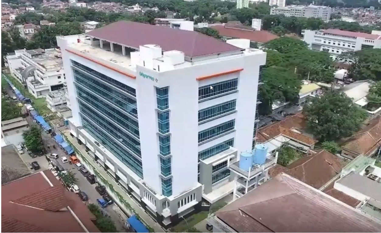
Figure 2: Photography of Building No. 43, Pasteur site, Bandung
