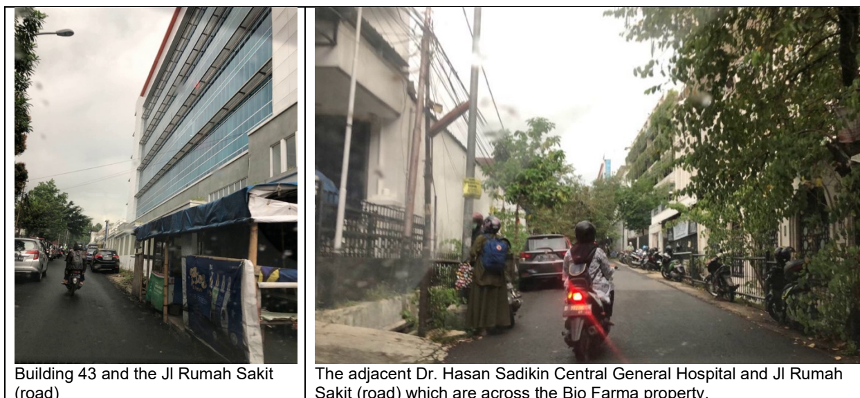
Figure 18: Photos of the adjacent road and hospital across Building 43
