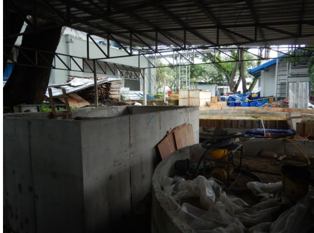
Figure 24: Third wastewater treatment facility under construction/installation in Bio Farma's Pasteur Site
