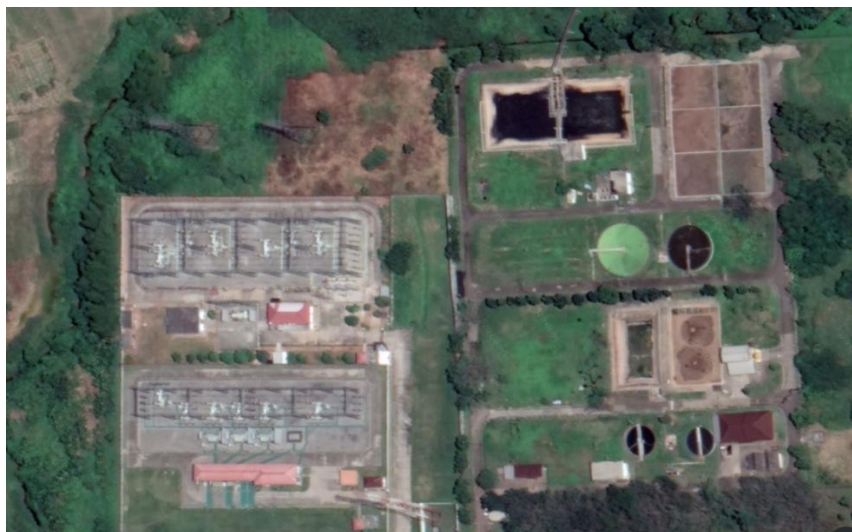
Figure 31: Wastewater treatment plant in Indotaisei Industrial Park
