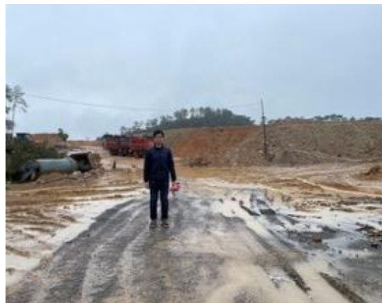
Current status of the site
