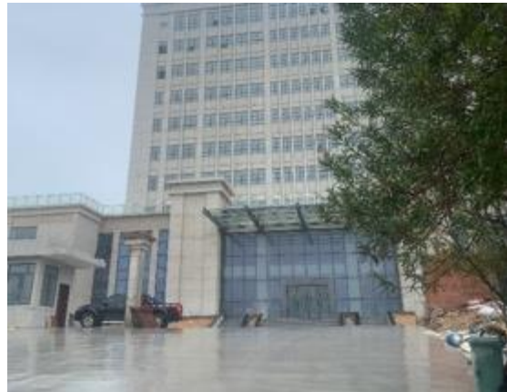
Cultural Palace for Workers of South China Federation of Trade Unions (under construction)
