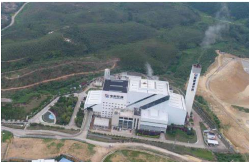
Figure III-6: Fangchenggang waste to energy incineration plant
