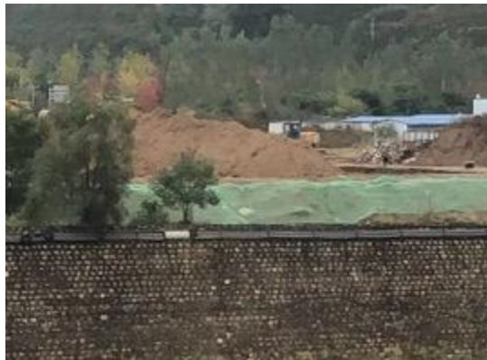
Vacant land in the west
