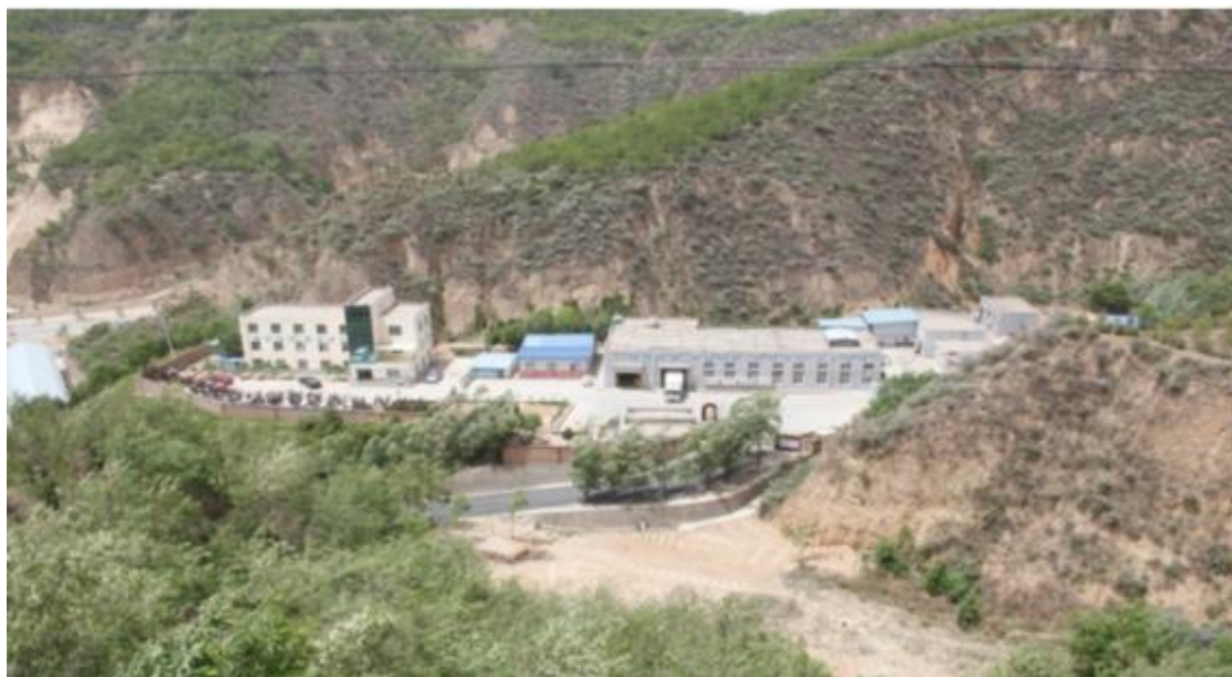
Figure III-8: Yan'an Shengyuan Medical Waste Disposal Center
