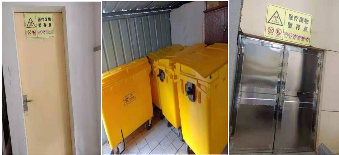
Figure 2-5 Existing medical waste storage point of Yan'an University Affiliated Hospital
