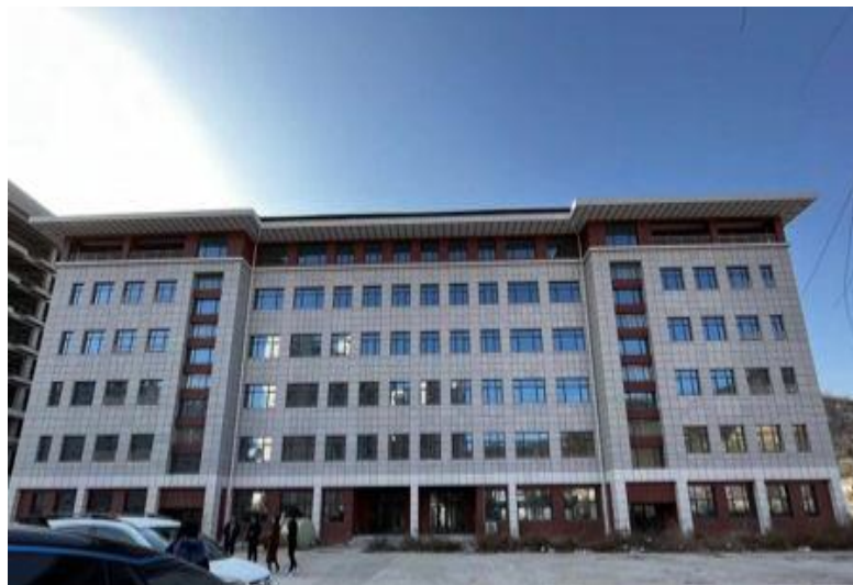
Figure 2-3 The part of the built facility available to the Sub-project
