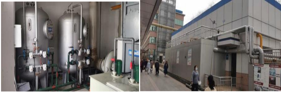
Figure 2-4 Existing sewage treatment station of the Yan'an University Affiliated Hospital
