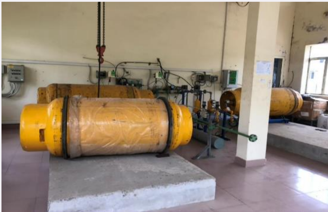
Photo 14: The existing chlorine gas storage house at the WTP
