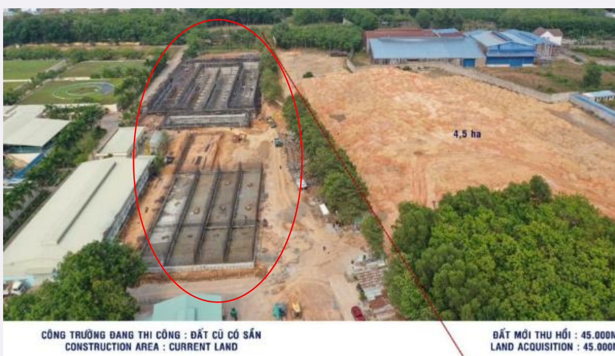
Photo 6: The existing water treatment facilities (left), the Project in the middle (in red oblong) and the Phase 2 expansion on the recently acquired land (right)
