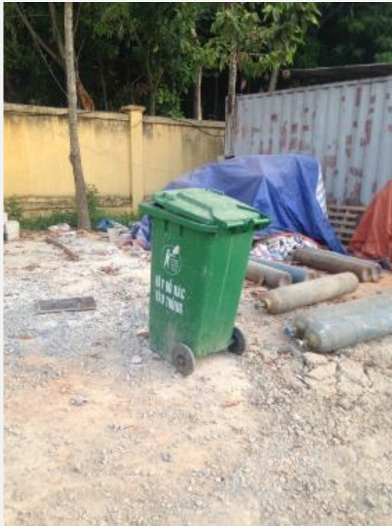
Photo 19: Oxygen cylinders on the ground at the construction site at the WTP
