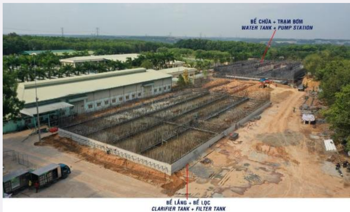
Photo 4: A view of the clarification tank and filtration tank of the Phase 1 expansion
