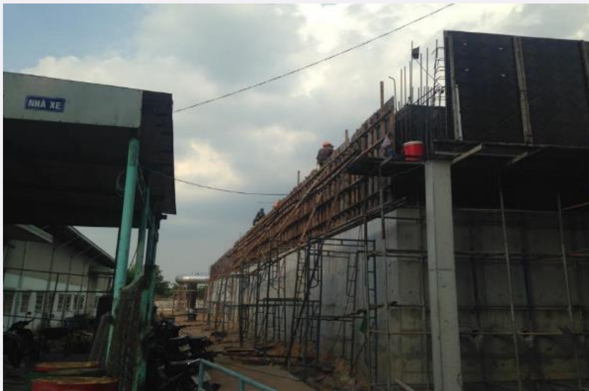
Photo 20: Workers working at high without harnesses at the construction site of the WTP.
