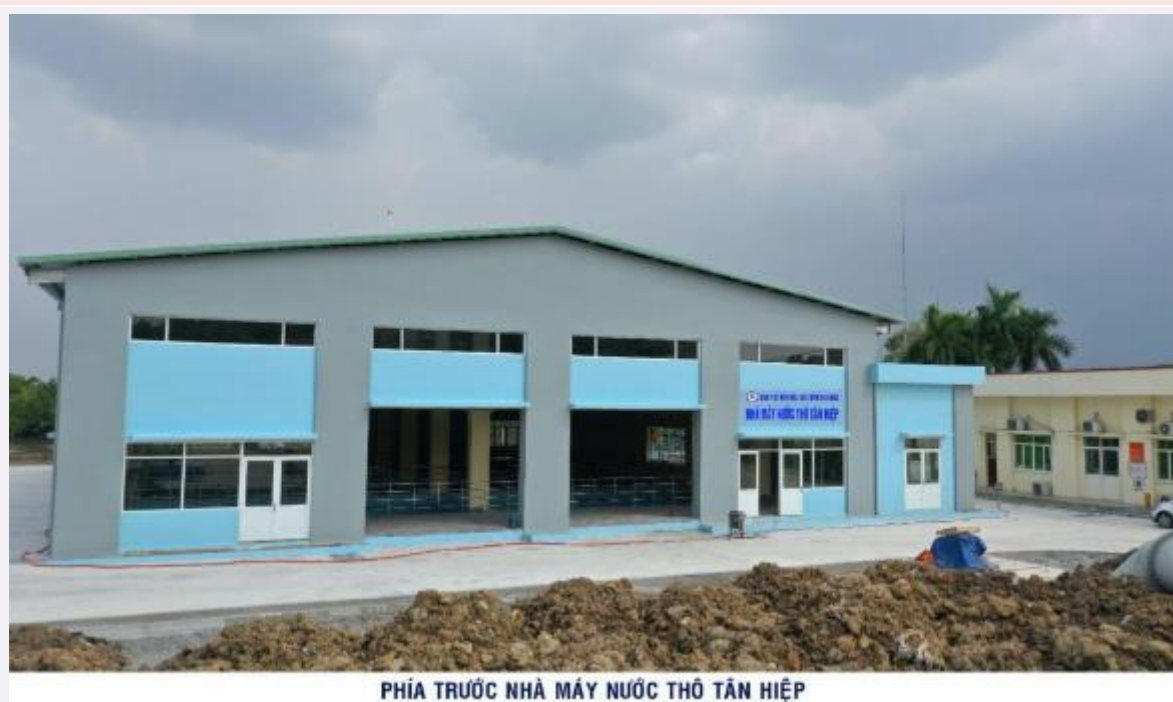
Photo 2: The front view of the Intake Station (photo taken in April 2020 by BIWASE)
