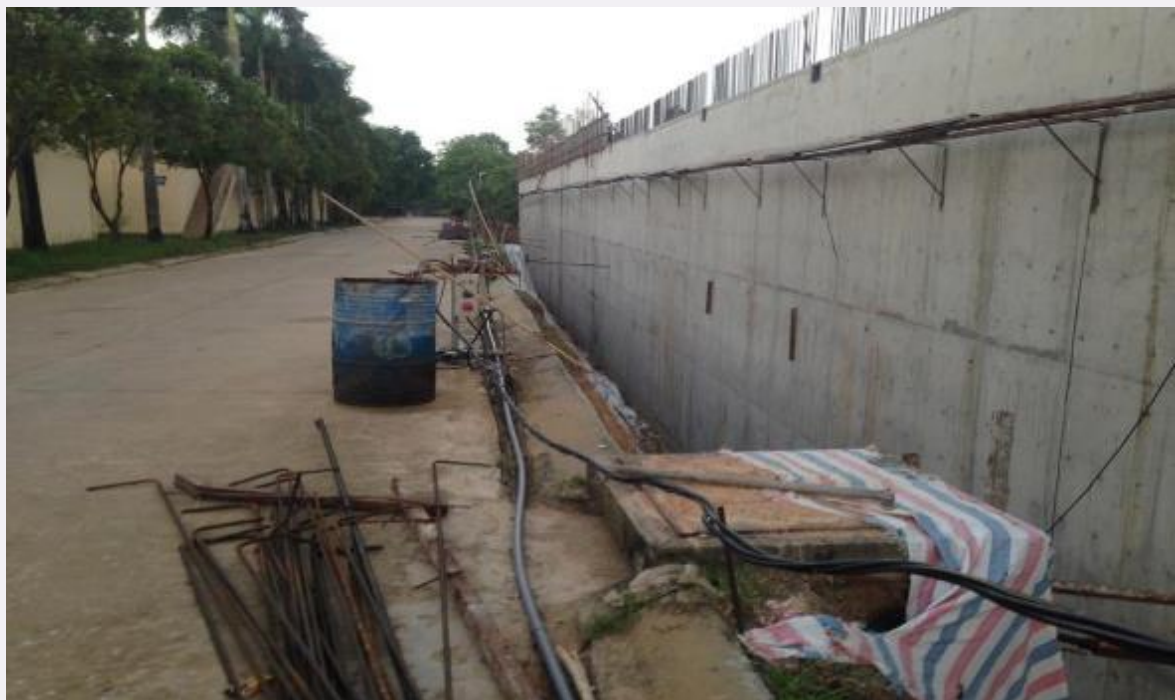
Photo 22: Construction site of the WTP without barricades and hazard warning signs
