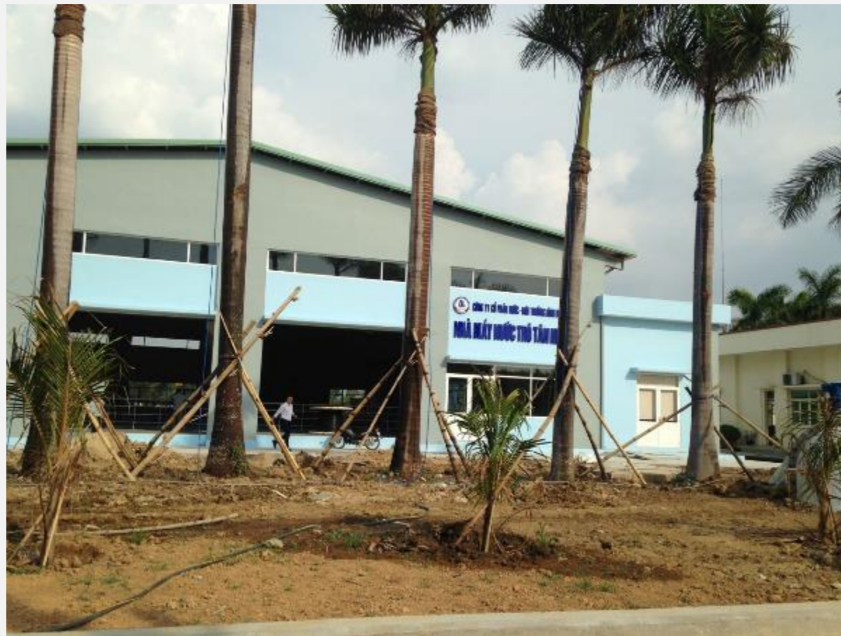
Photo 3: A view of the Intake Station at the time of the site visit in May 2020
