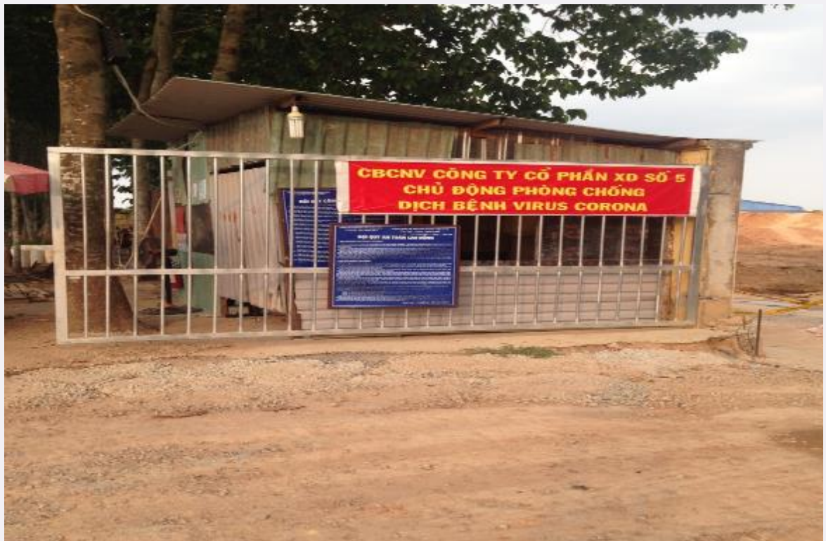
Photo 21: Entrance to the construction site at the WTP with construction safety notes and banners for COVID 19 prevention
