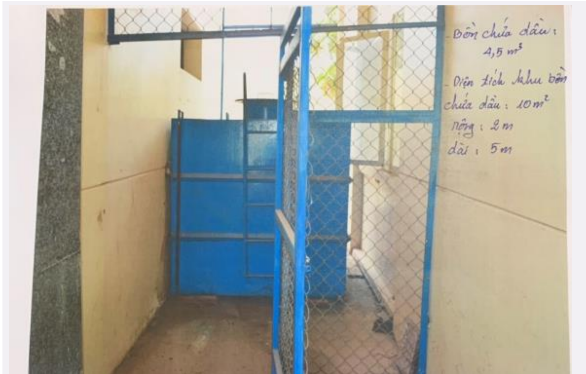
Photo 9: A diesel storage tank at the WTP
