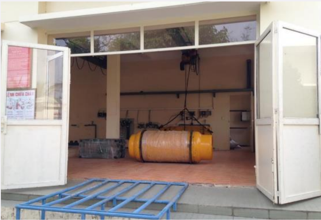
Photo 12: The existing chlorine gas storage house at the Intake Station
