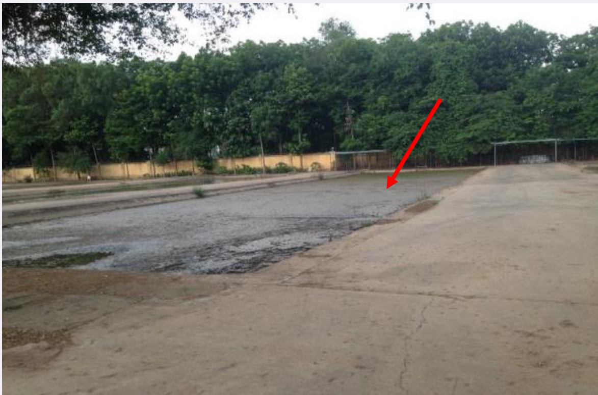
Photo 24: Existing sludge drying yard in the WTP
