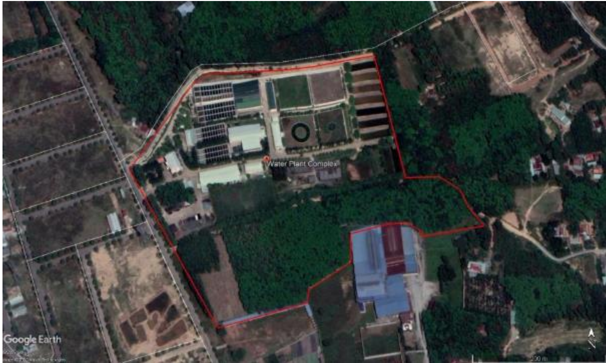
Figure 2-1 Aerial Imagery of Tan Hiep Water Treatment Plant as of February 2018
