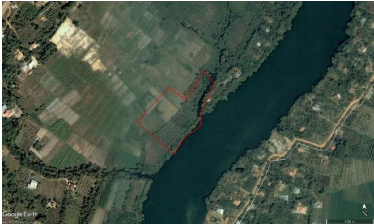
Figure 2-12 Historical Aerial Imagery of the Intake Station Dated in December 2003
