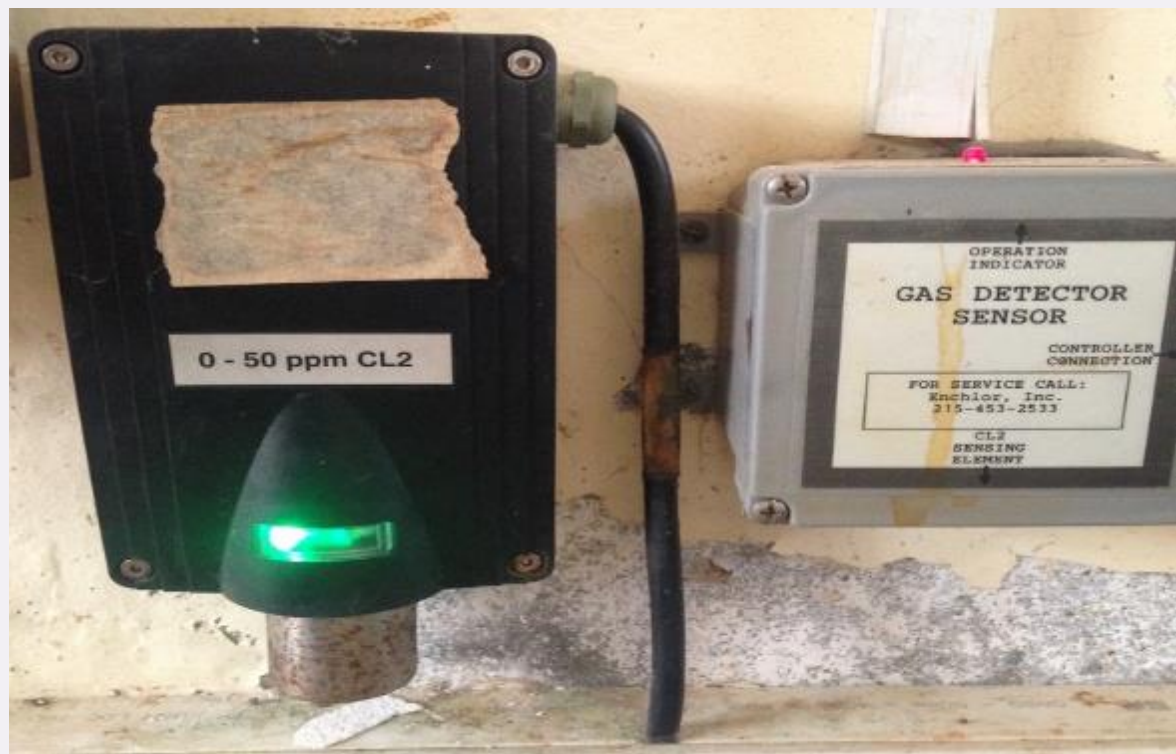
Photo 17: A chlorine gas detector system in the existing chlorine house at the WTP
