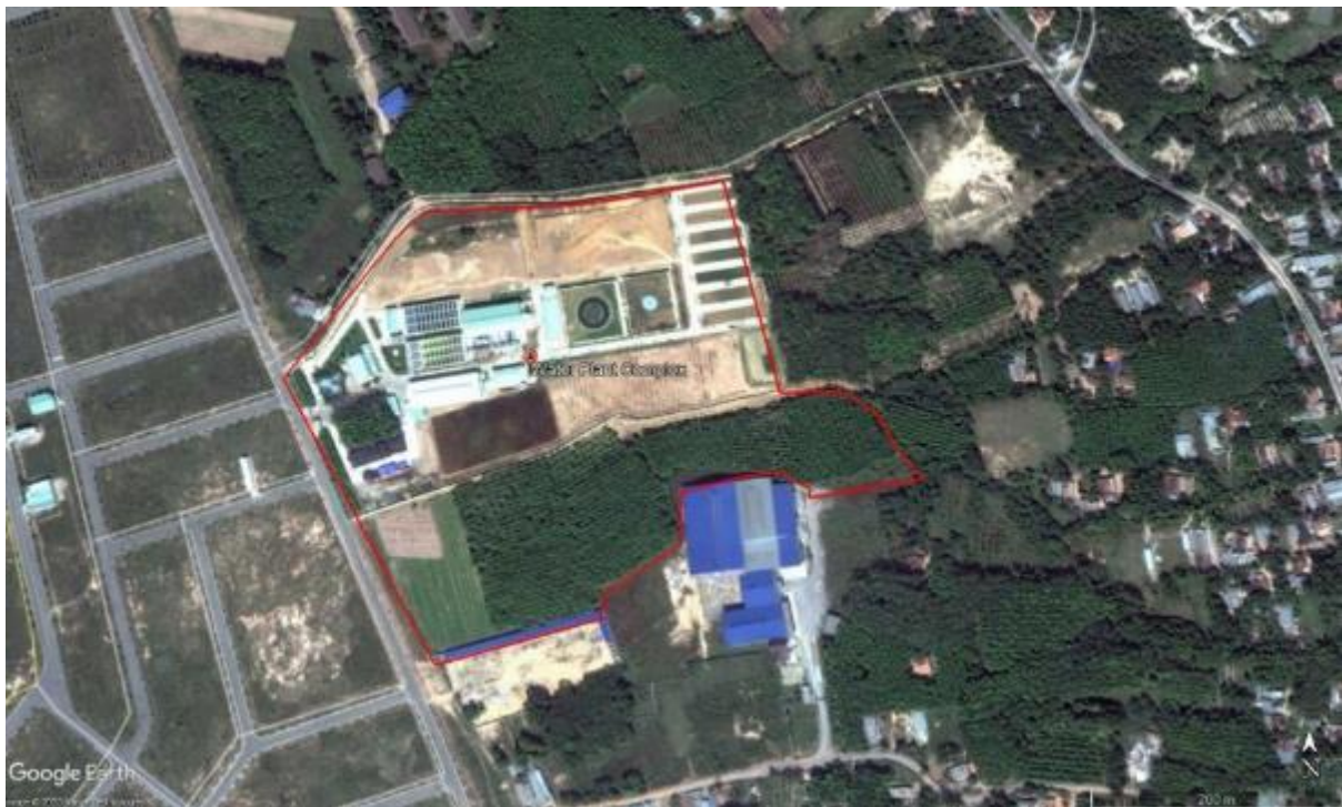
Figure 2-4 Aerial Imagery of Tan Hiep Water Treatment Plant in December 2010
