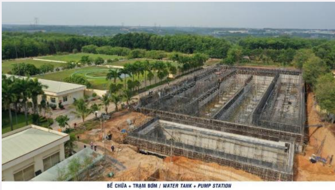
Photo 5: A view of the water tank and pump station of the Phase 1 expansion Project under construction
