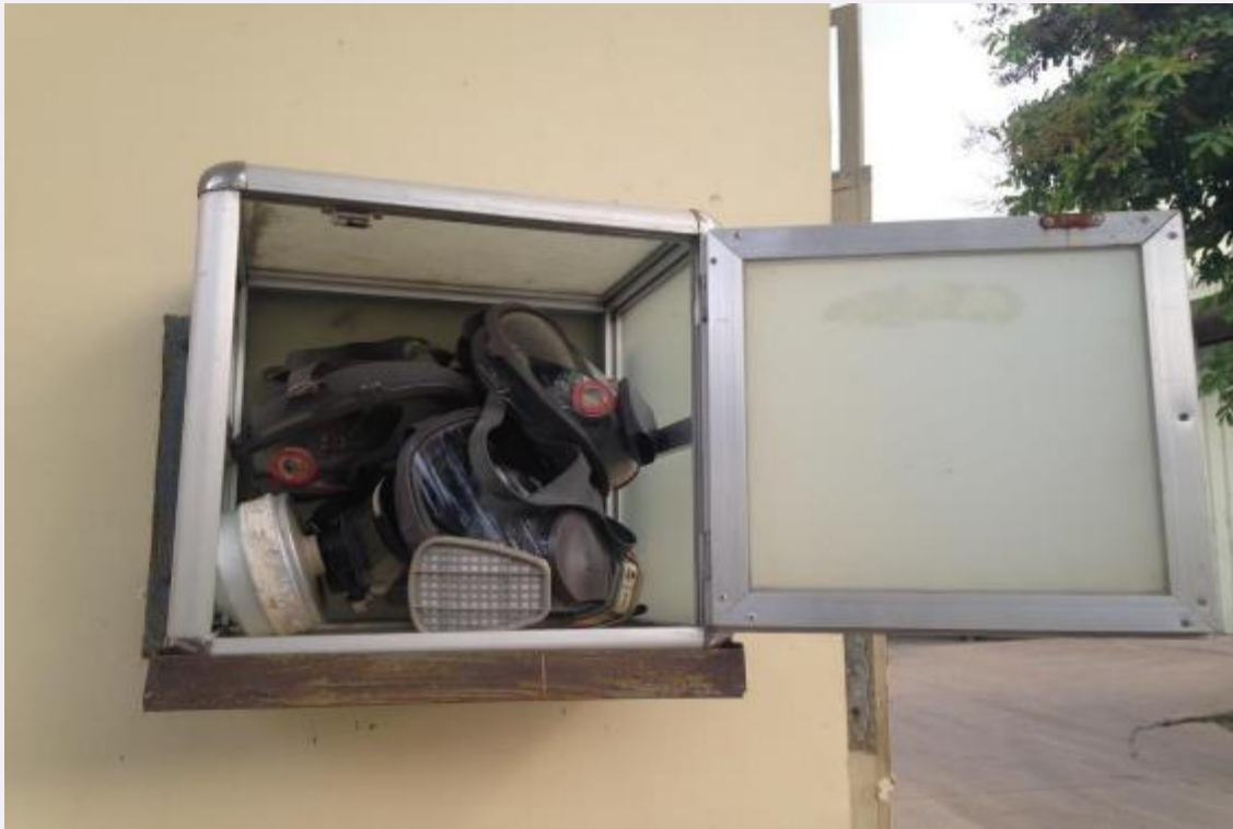
Photo 15: Respirators stored in a box outside of the existing chlorine house at the WTP
