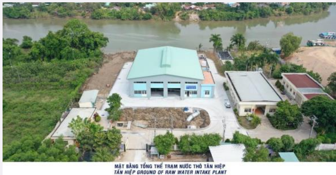
Photo 1: The raw water intake station (photo taken in April 2020 by BIWASE)
