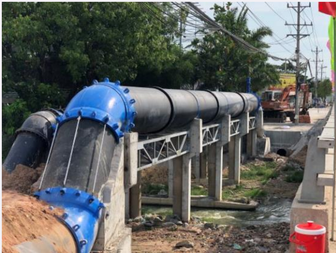
Photo 10: A section of the raw water transmission pipeline of Tan Hiep WTP
