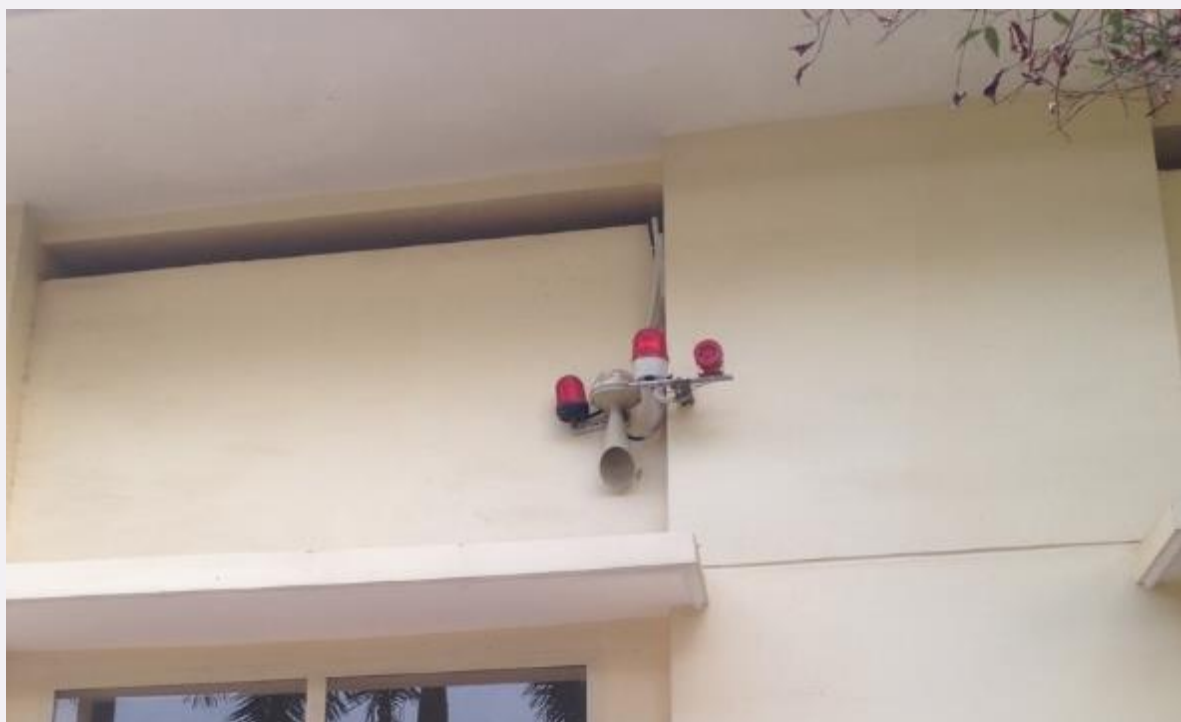
Photo 16: A chlorine gas leak warning alarm and bell installed at the existing chlorine gas house of the WTP
