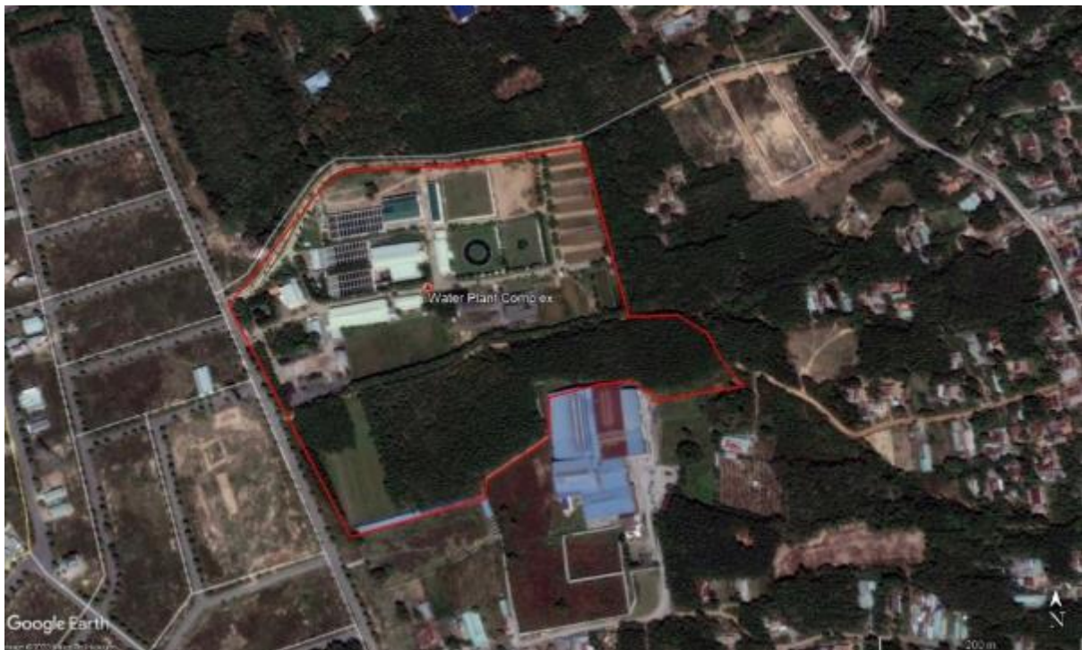
Figure 2-6 Aerial Imagery of Tan Hiep Water Treatment Plant in January 2017
