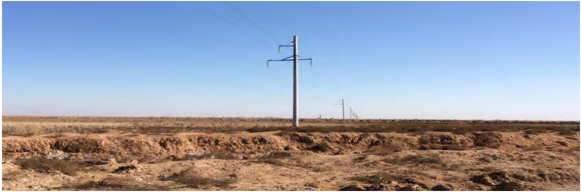
Figure 18 Existing 100 kV transmission line transect from the site
