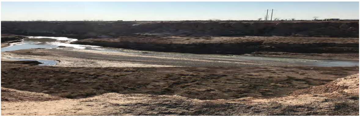
Figure 19 New 220 kV transmission line – river Karasu crossing (width 12.4 meters)
