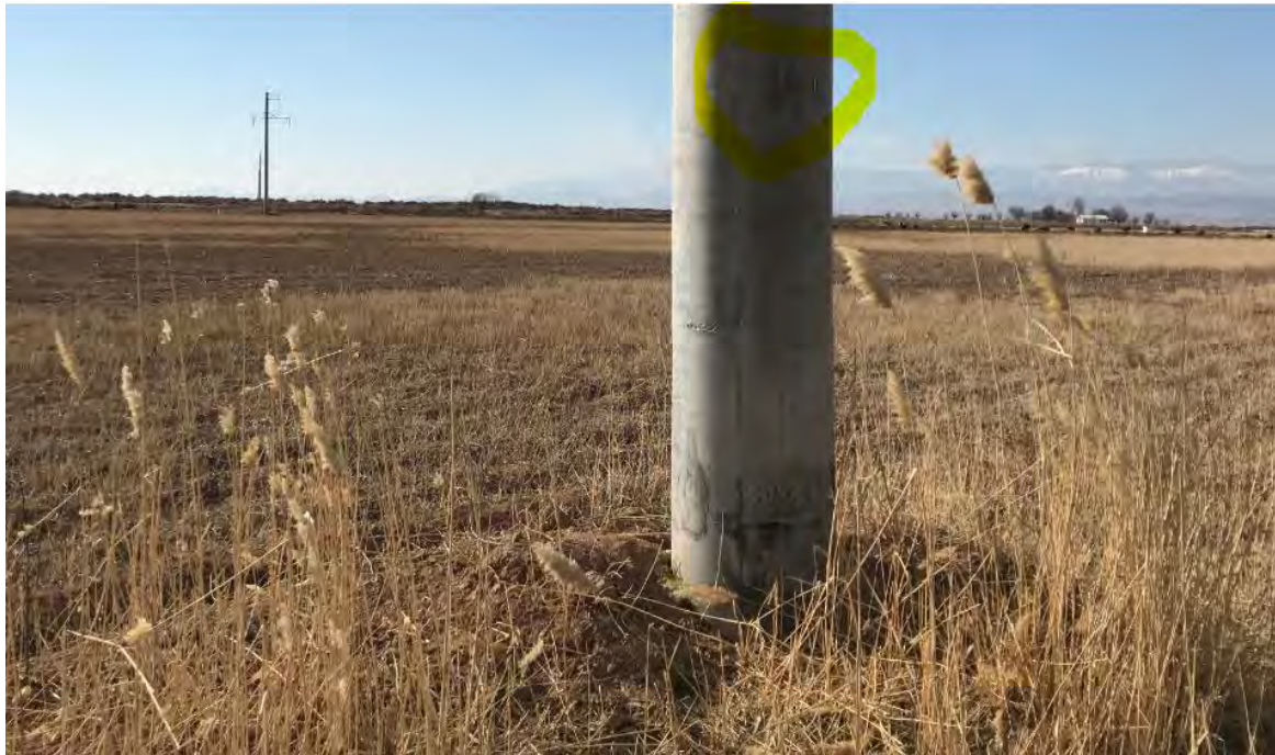
The numbers of towers before the M39 are 144 and 143, after the M39.
