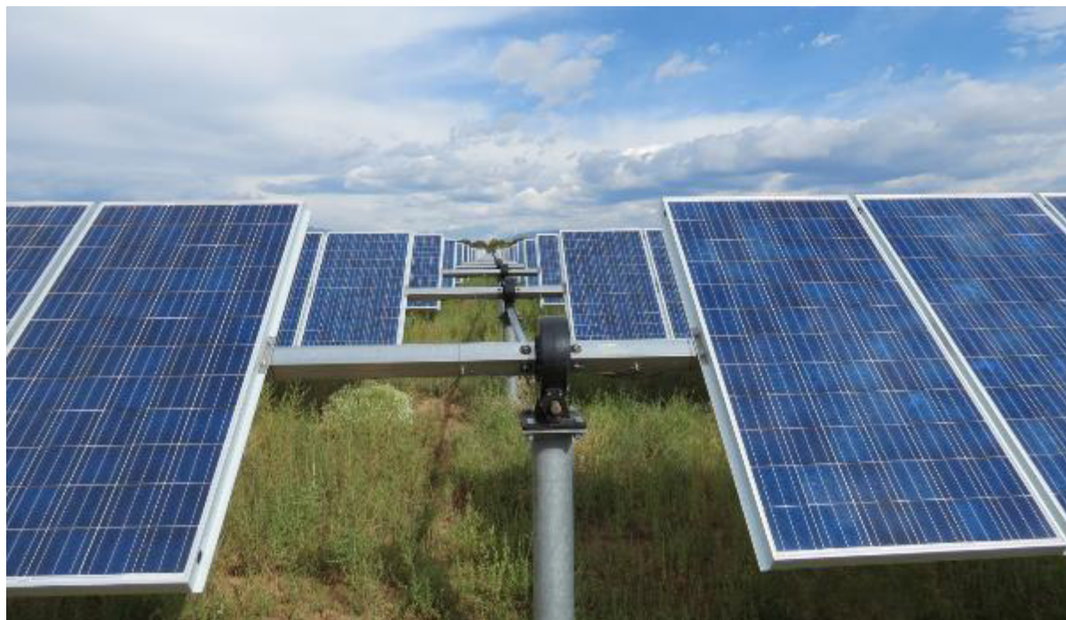
Figure 2-13: Typical PV Facility, using Tracking System
