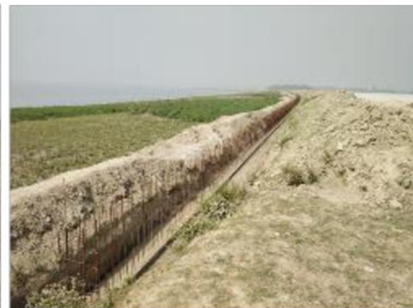
Retention wall (boundary wall) under construction along the western boundary of Site
