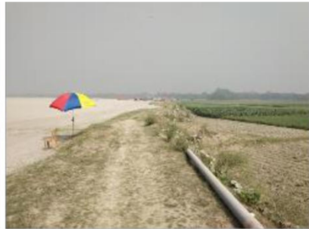
Relative elevation difference between raised surface level of Site and natural ground level
