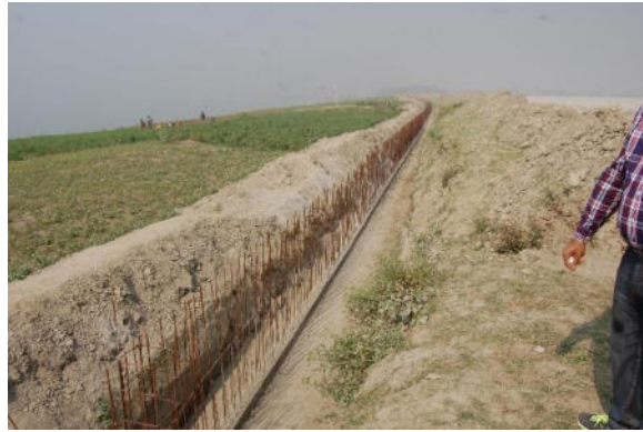
Construction of retaining wall (ongoing)
